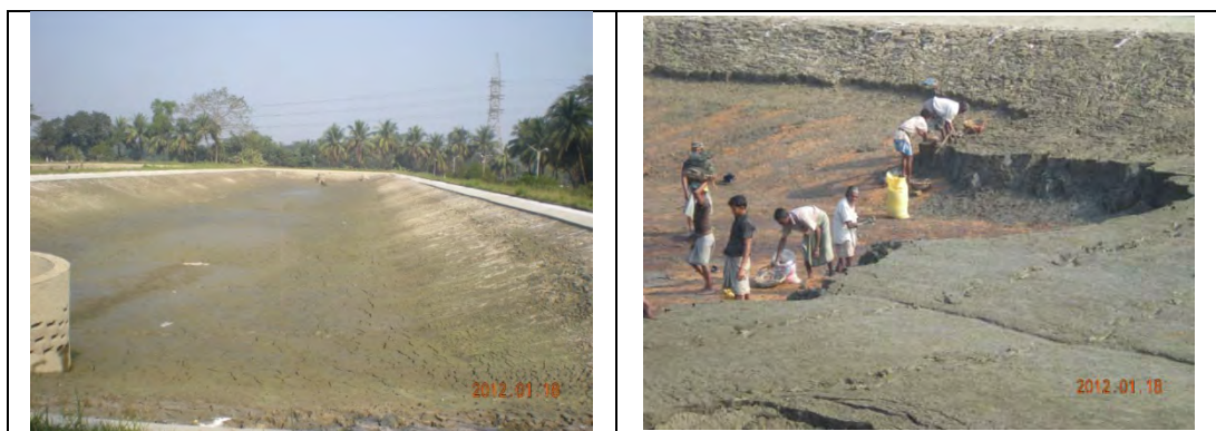
Figure 7.7.4 Pictures on Removal of Sludge at Mohara WTP (18/1/2012)
