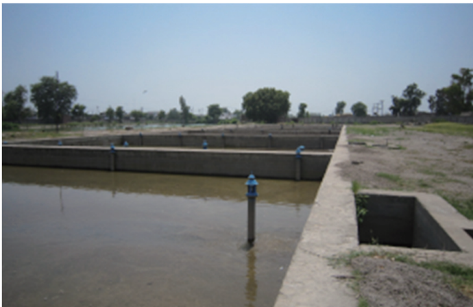
Existing slow sand filtration at Jhal Khanuana WTP
