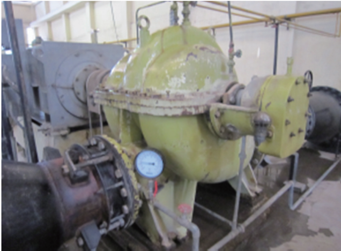
Aged distribution pump installed in 1991 in Terminal Reservoir
