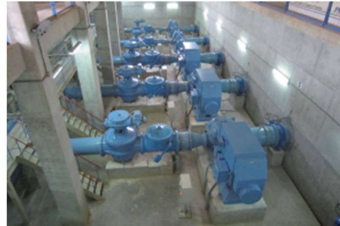
Newly completed distribution pumps in Terminal Reservoir by JICA grant aid
