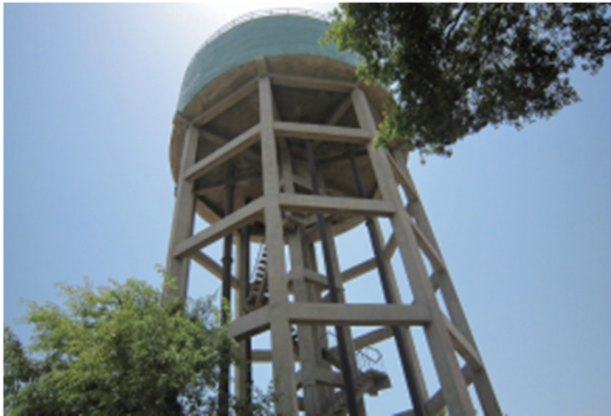
Elevated Tank in the city
