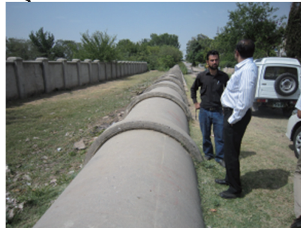
Aged malfunctioning water transmission pipe
