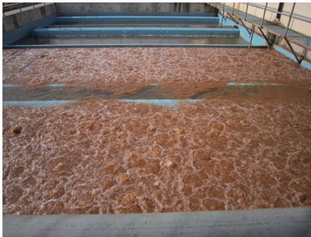
Filter back-washing in Rawal WTP
