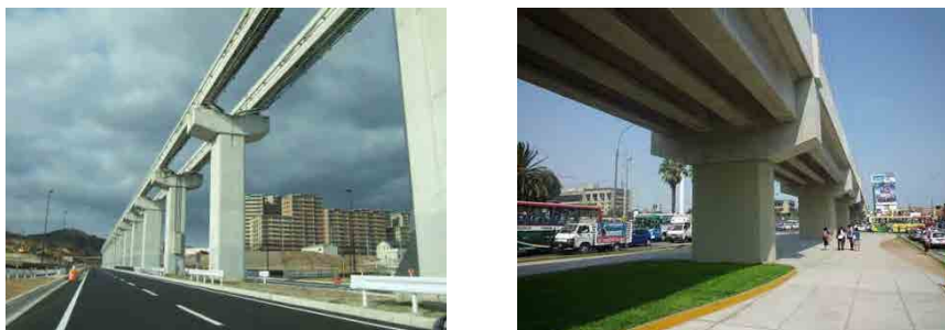
Figure 6.12 Monorail's Superstructure and Conventional Slab Structure
