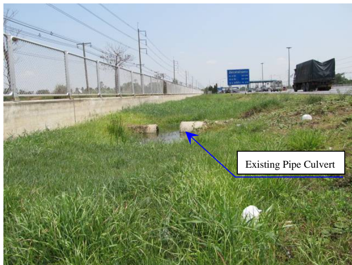
Photo 2-2-1-2.2 Condition of Existing Drainage Facility
