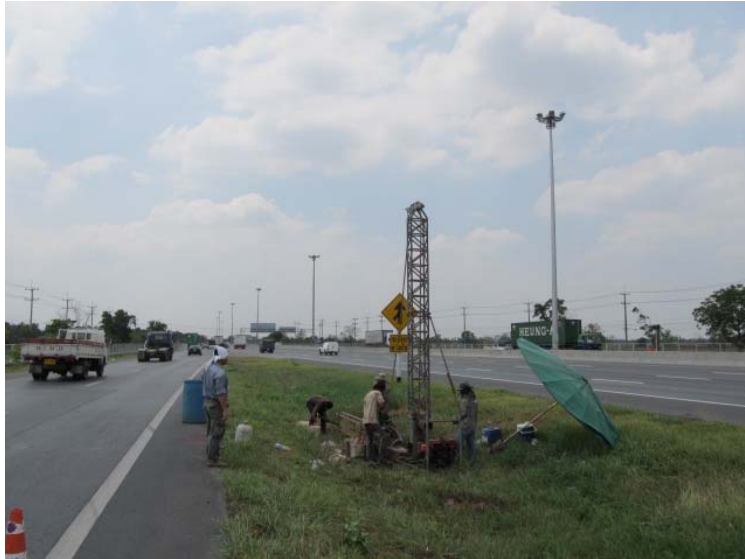
Photo 2-2-1-2.1 Drilling Work in Progress
