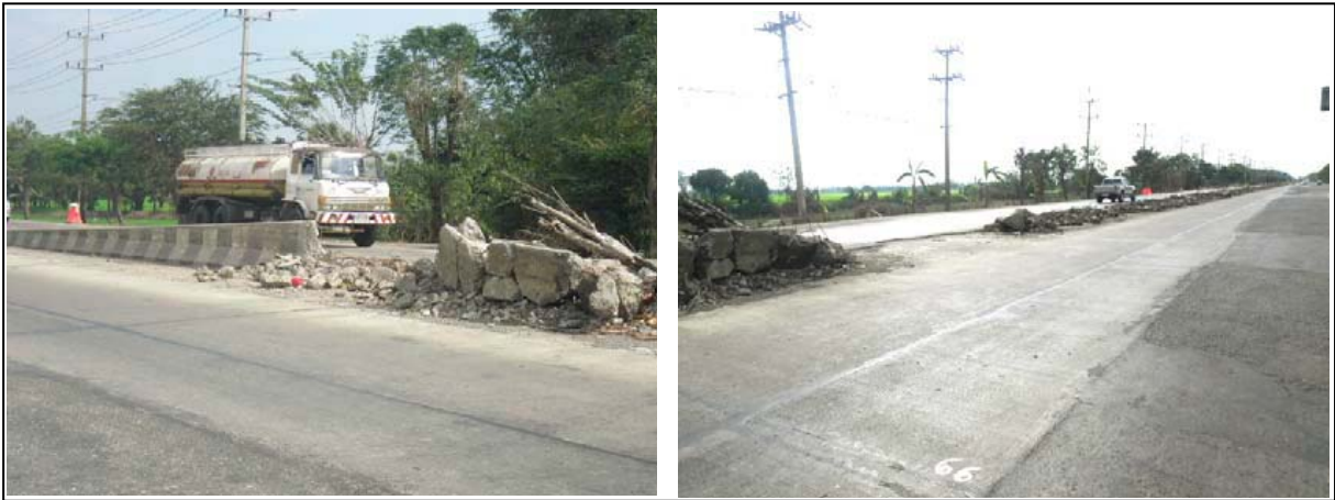
Photo 1-2.1 Demolition Condition of Concrete Barrier on the Median of NR-1
