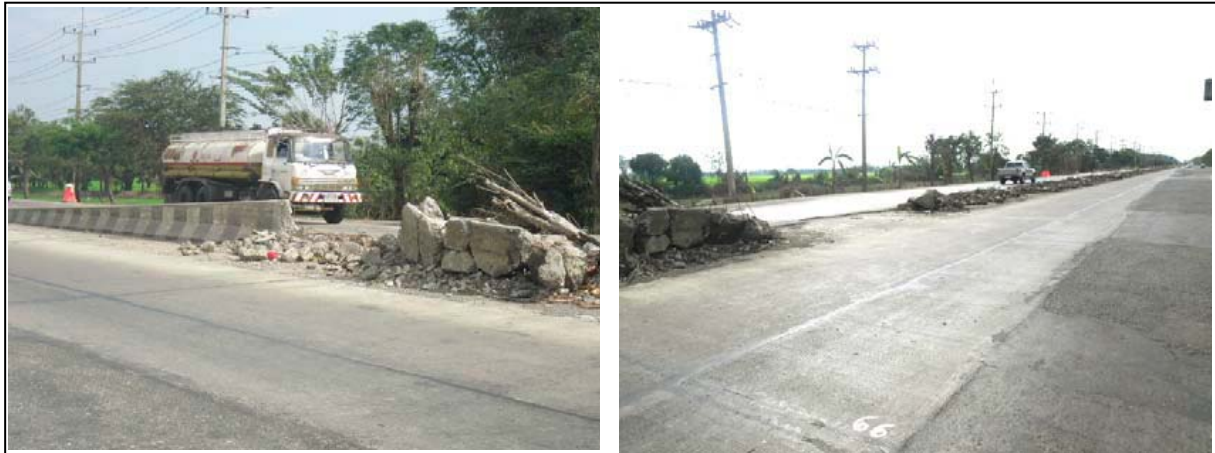
Photo 2-2-1-3.1 Demolition Condition of Concrete Barrier on the Median of NR-1
