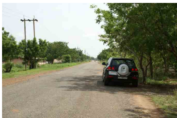
Photo 3-5 Existing Road Passes through the community
