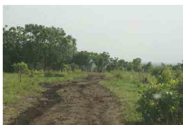
Photo 3-21 Condition of Track (1)
