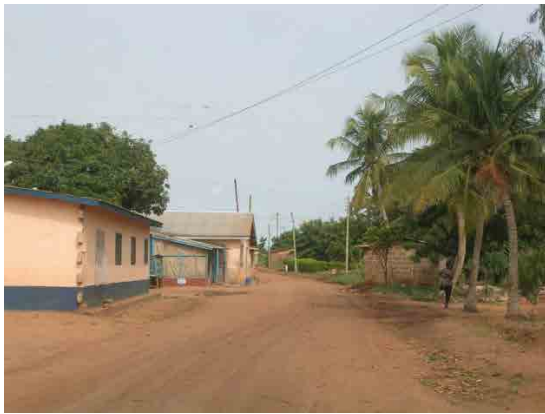
Photo 3-11 Houses Encroaching Existing Road at Aveyime
