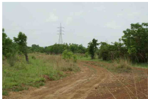
Photo 3-22 High Voltage Cable and Track to Adidome
