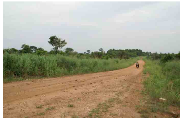
Photo 3-18 Rehabilitated Feeder Road near Frankadua
