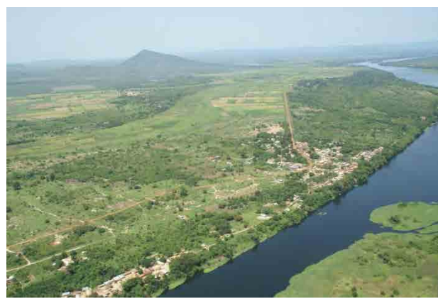
Photo 3-9 Road Alignment in Volivo
