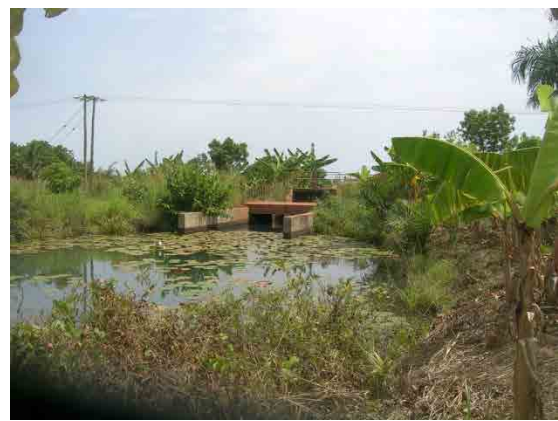
Photo 3-8 Unused Irrigation Canal at Asutsuare
