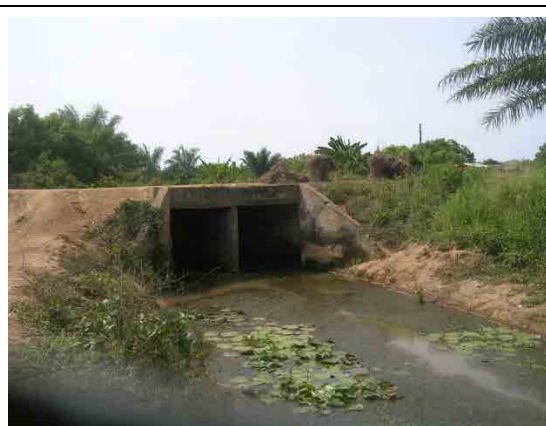
Photo 3-10 Box Culvert at Lukpe River
