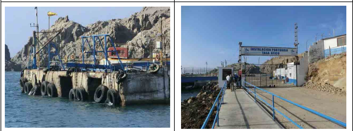
Foundation of Install Area
