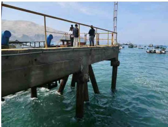
Foundation of Install Area
