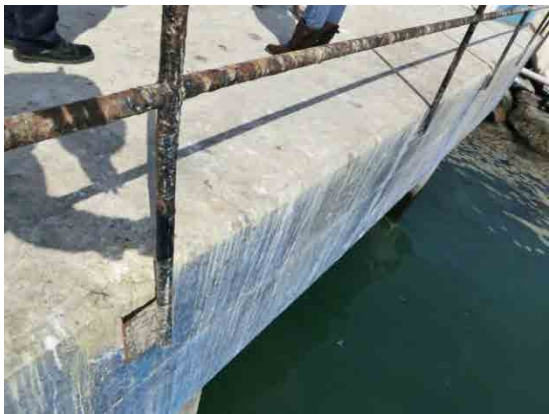
Foundation of Install Area
