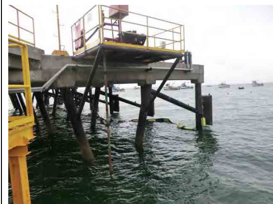
Foundation of Install Area
