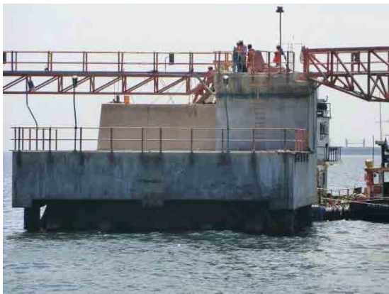
Foundation of Install Area
