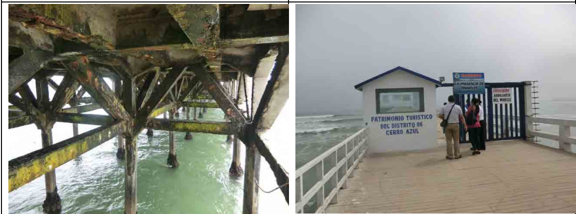
Foundation of Install Area
