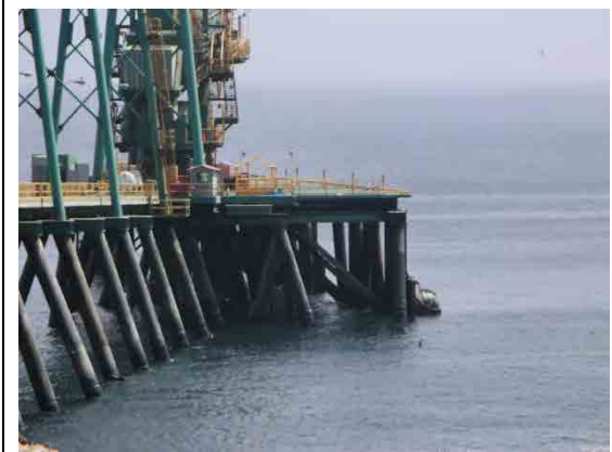
Foundation of Install Area
