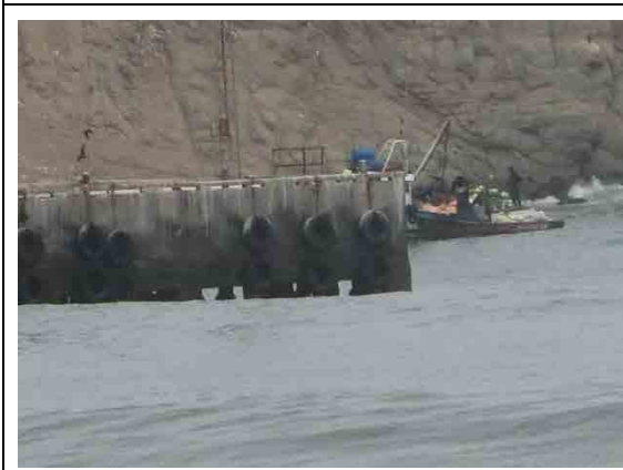
Foundation of Install Area
