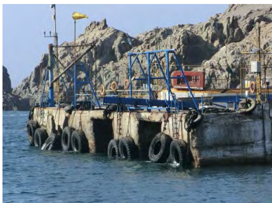
Foundation of Install Area
