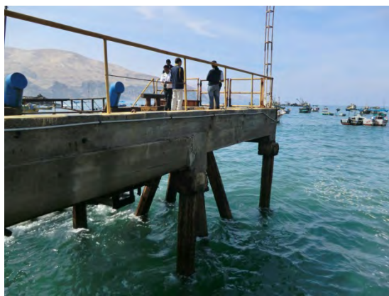
Foundation of Install Area
