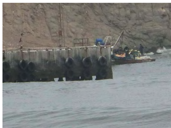
Foundation of Install Area
