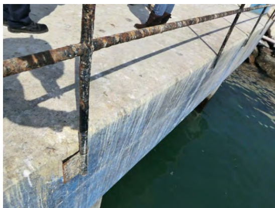
Foundation of Install Area
