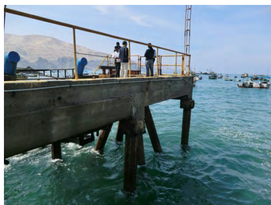
Foundation of Install Area
