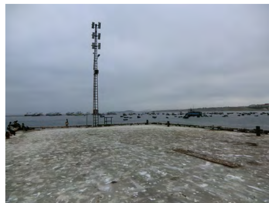
Install Area of Tide Observation System
