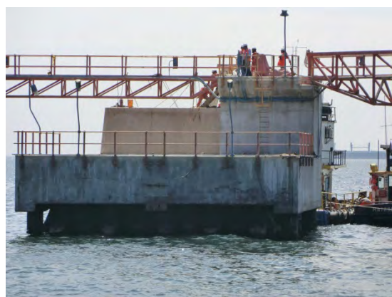
Foundation of Install Area
