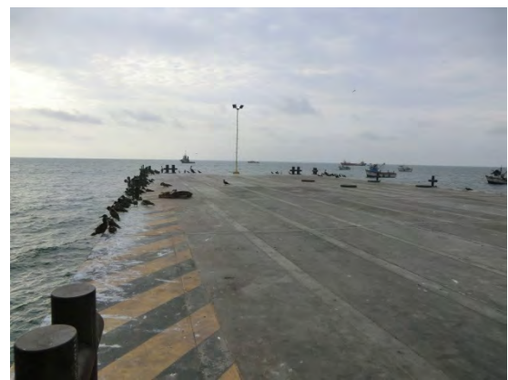
Install Area of Tide Observation System
