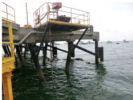
Foundation of Install Area
