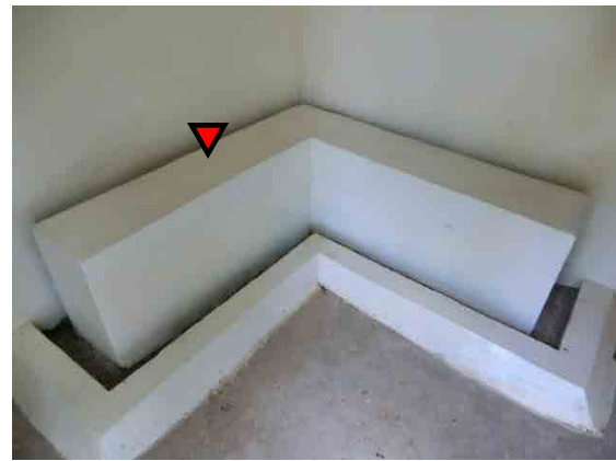
Install Area of Accelerometer
