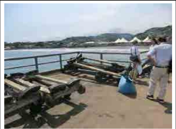
Install Area of Tide Observation System
