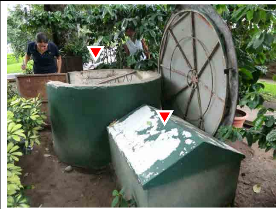
Install Area of Accelerometer
