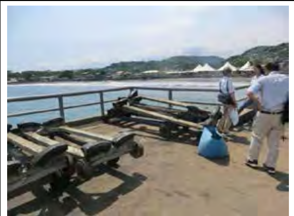
Install Area of Tide Observation System
