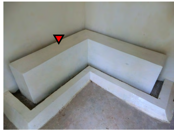
Install Area of Accelerometer
