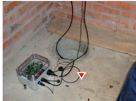
Install Area of Broadband Seismometer
