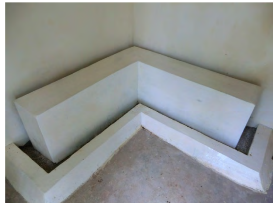
Install position of Seismometer
