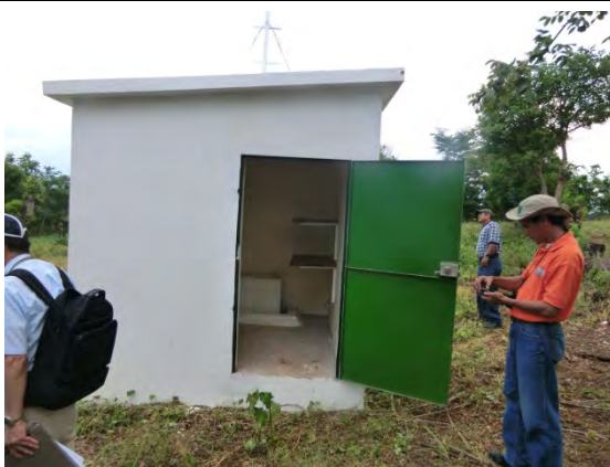
Install position of GPS sensor
