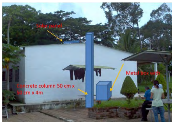
Install position of GPS sensor 2
