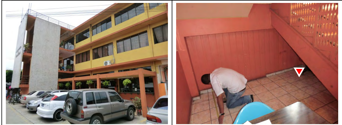
Building of Alcaldía de Quezaltepeque
