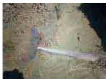
Cracks due to heavy traffic load
