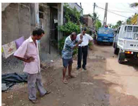
Borella Leak Detection (Confirmation survey)
