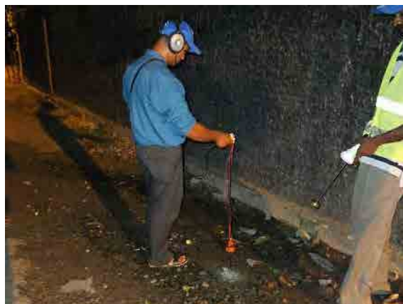
Activity of Pilot Project (Leakage Detection in Night Survey)
