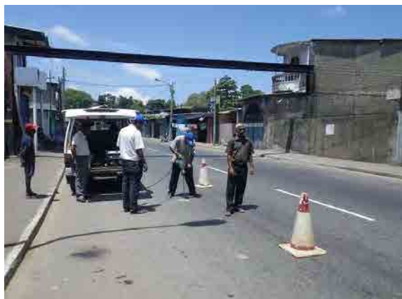
Activity of Pilot Project (Kotahena) (Excavating Leakage Point)
