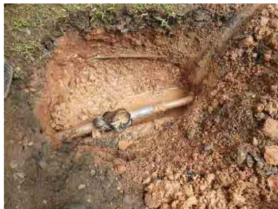
Activity of Pilot Project (Kotahena) (Exposing Leaking Pipe)
