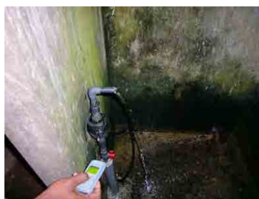
Kotahena Meter Installation to Free Water Outlet
