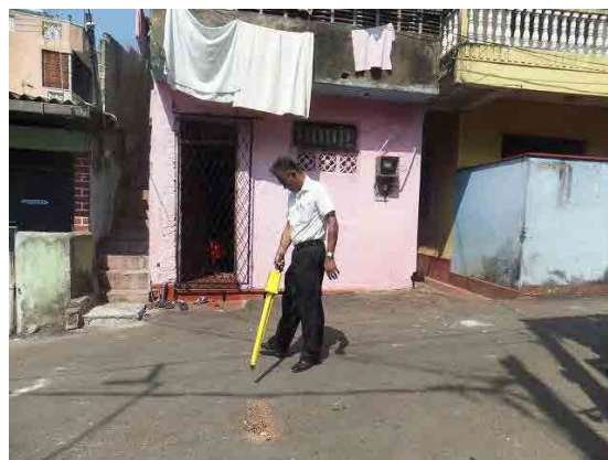
Activity of Pilot Project (Kotahena) (Leak Detection)
