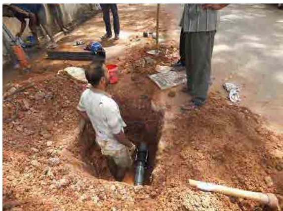
Activity of Pilot Project (Borella) (Leak Repair)
