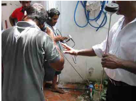
Borella Leak Detection (Acoustic Survey)
