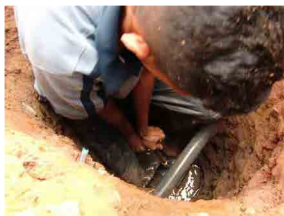
Borella Installation of New Service Connection
