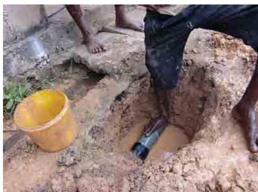
Borella Leak Repair Work
