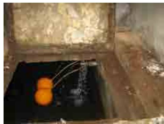
Activity of Pilot Project (Borella) (Repairing Float Valve of Sump for Condominium)
