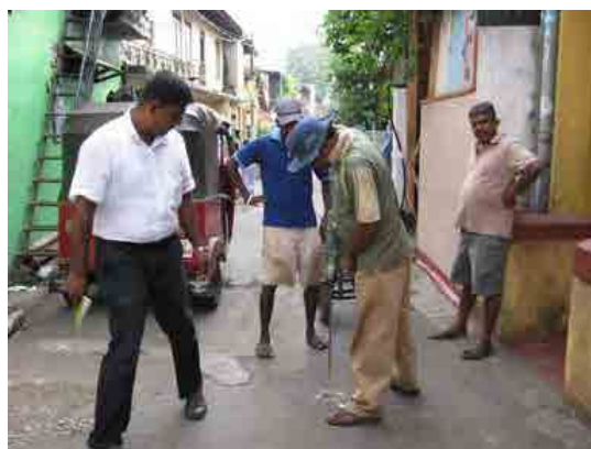
Kotahena Leak Detection (Pinpoint Survey)
