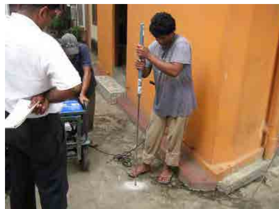
Kotahena Leak Detection (Pinpoint Survey)
