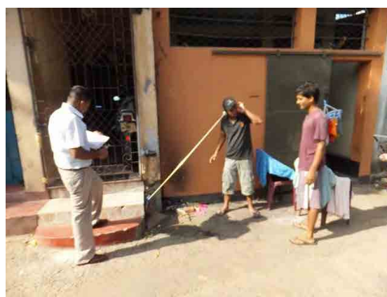
Activity of Pilot Project (Borella) (Leak Detection)
