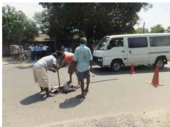
Activity of Pilot Project (Kotahena) (Hydraulic Isolation of Sub-zone)
