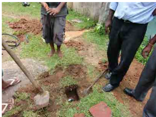
Borella Searching Buried Customer Meter (Excavating buried meter)
