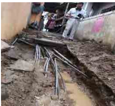
Activity of Pilot Project (Kotahena) (Bundle Pipe Replacement (1))
