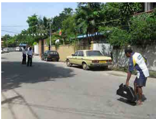
Borella Tracing of Buried Pipe
