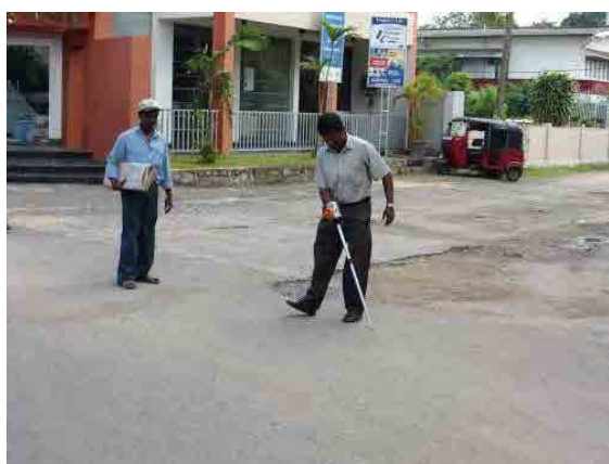
Kotahena Valve Locating
