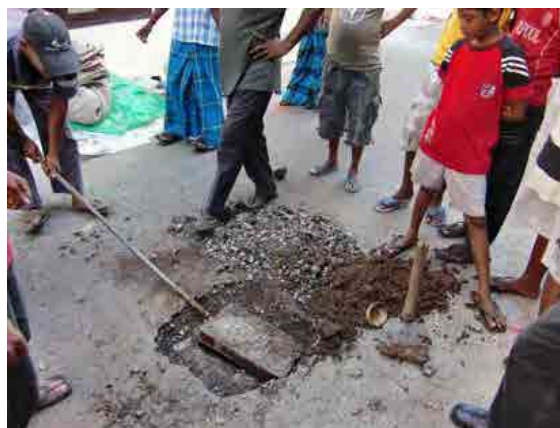
Kotahena Valve Locating
