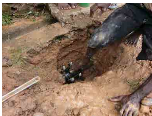
Borella Leak Repair Work
