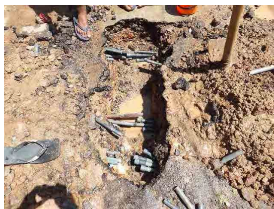
Activity of Pilot Project (Kotahena) (Bundle Pipe Replacement (2))
