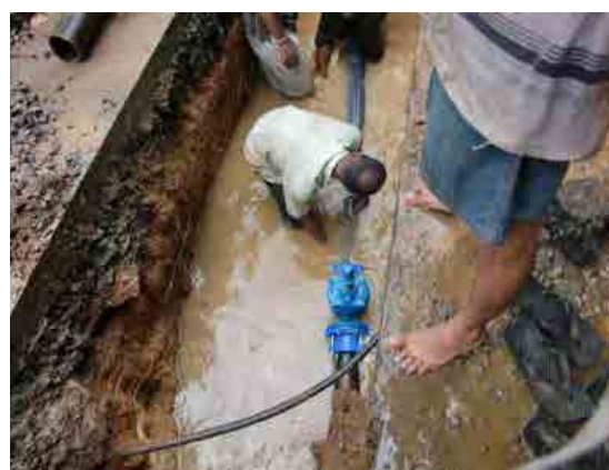
Borella Valve Installation
