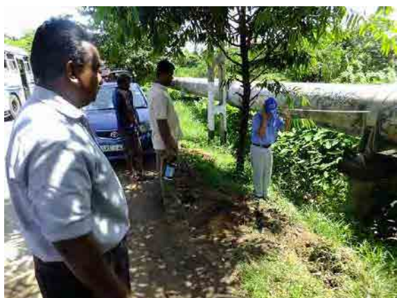
Activity of Pilot Project (Training on Leak Detection for Large Diameter Pipes (2))
