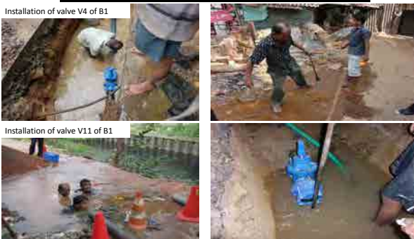
Installation of valve V4 of B1
