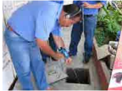
Contact the rod to the water meter
