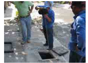
Listen to the noise at the customer meter
