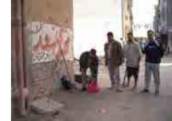
Set the transmitter on the pipe line
