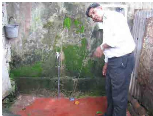
Kotahena 漏水調査 (Acoustic survey)
