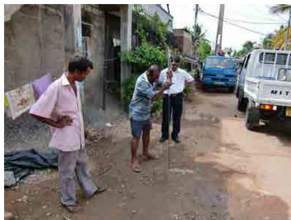
Borella 漏水調査 (Confirmation survey)
