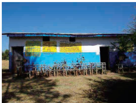
External view of an existing school building
