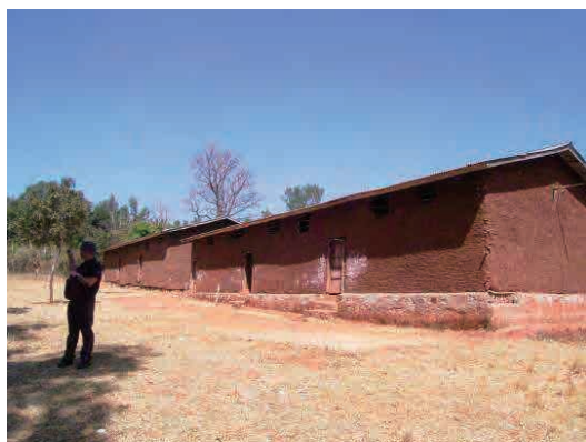
External view of existing buildings
