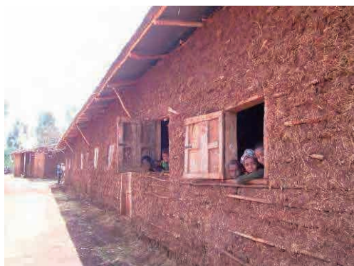
External view of existing buildings
