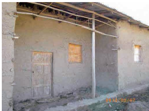
External view of an existing school building
