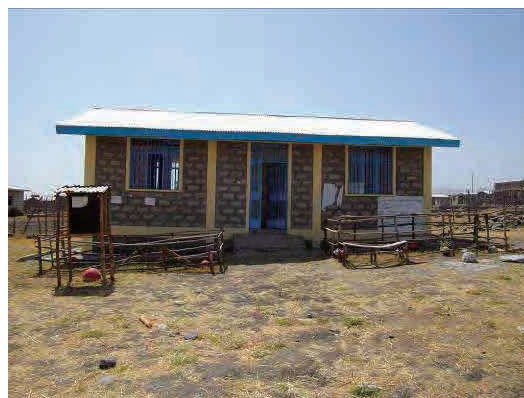
External view of an administration building
