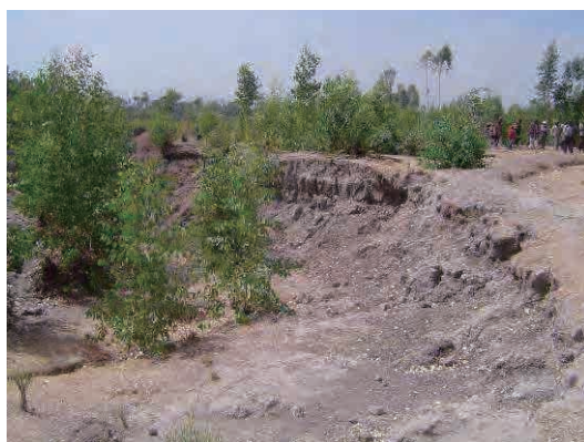
Back of the construction site
