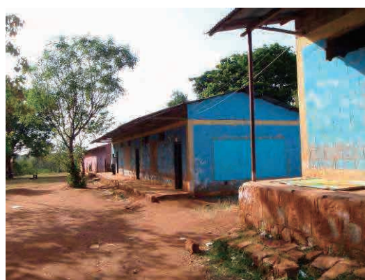
Buildings of Chichu secondary school in woreda capital
