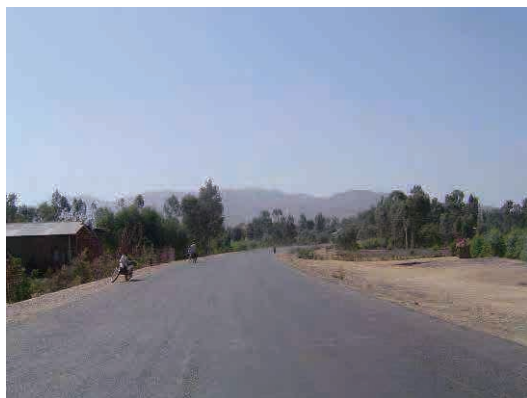
Frontal road of the construction site
