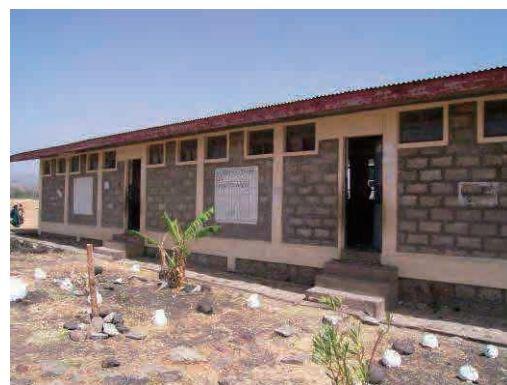
External view of an existing building
