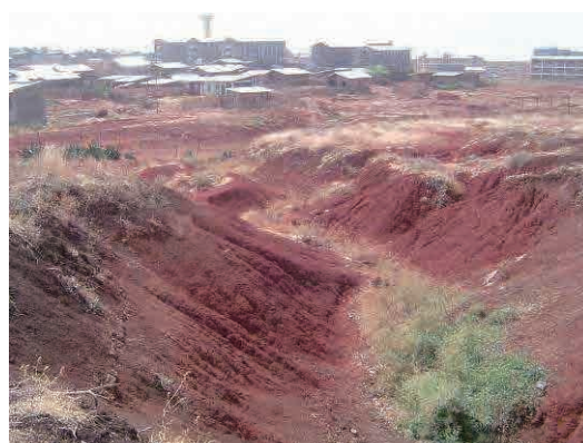
Back of the construction site
