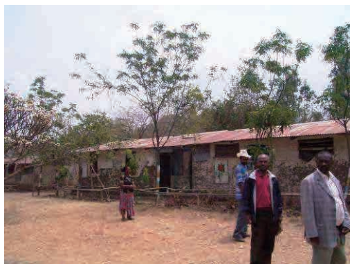
External view of an existing building
