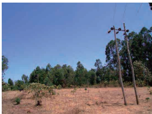
Power lines within the construction site
