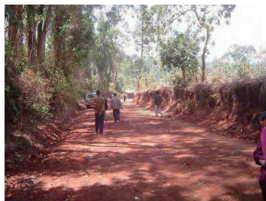
Side road of the construction site
