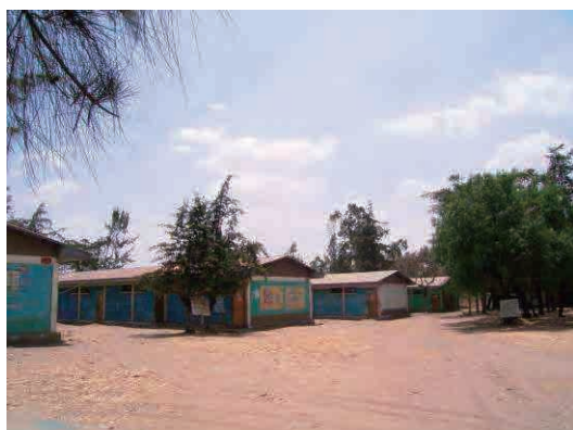
Existing buildings of Halaba secondary & preparatory school
