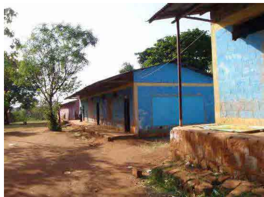
Buildings of Chichu secondary school in woreda capital
