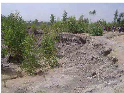
Back of the construction site
