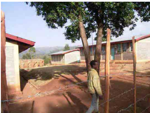
Adjacent primary school to the construction site
