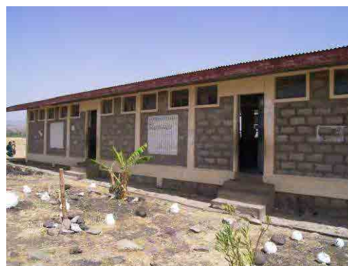
External view of an existing building
