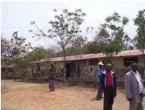
External view of an existing building
