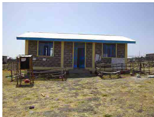
External view of an administration building
