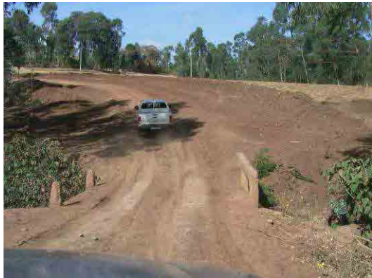
Access road to the construction site
