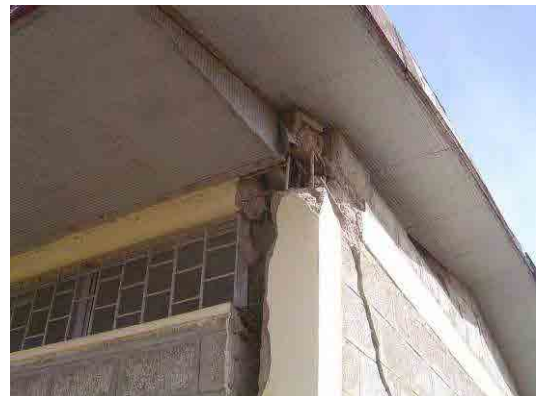
A damaged building by an earthquake <adjacent primary school to the site>
