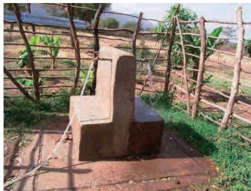
Water facility within the school compound
