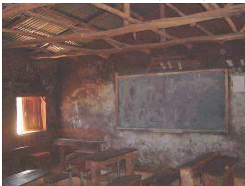
Inside of a classroom
