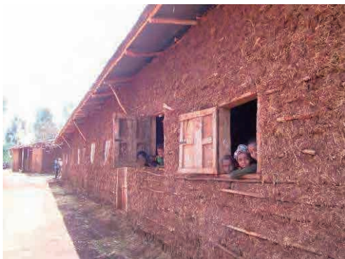
External view of existing buildings
