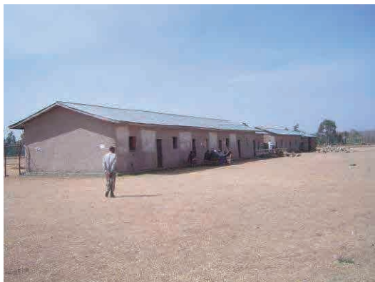
External view of existing school buildings
