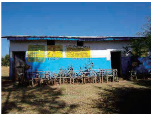
External view of an existing school building
