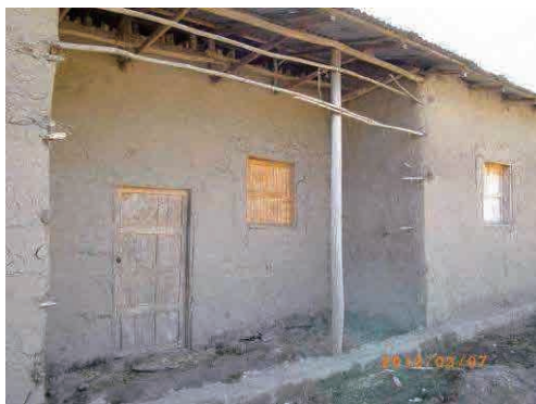
External view of an existing school building
