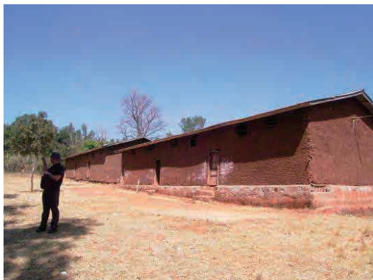
External view of existing buildings
