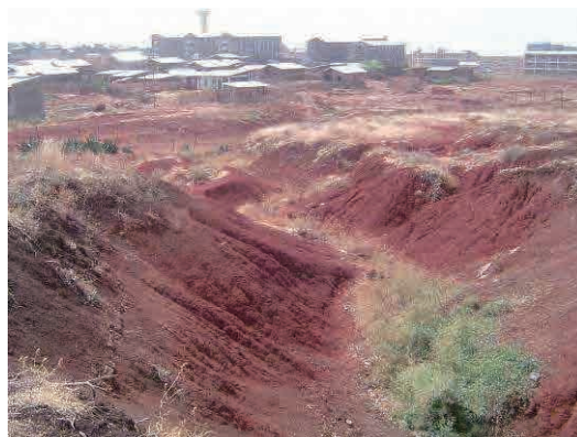
Back of the construction site
