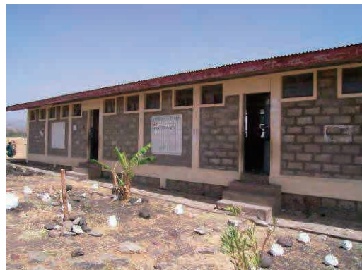
External view of an existing building
