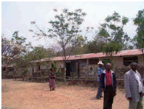
External view of an existing building
