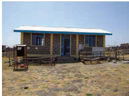
External view of an administration building
