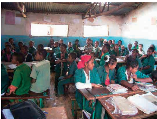
Inside of a classroom of the adjacent primary school (Currently, secondary students are using the room)
