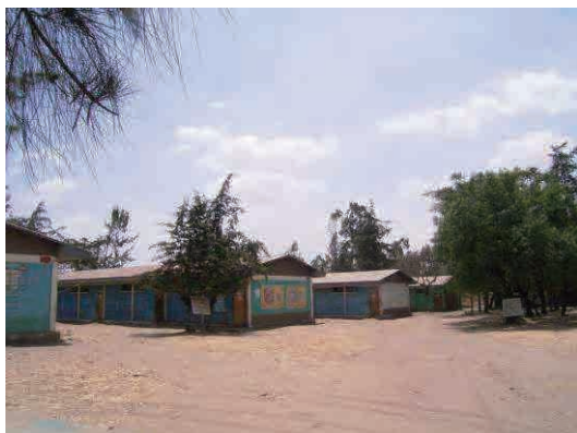
Existing buildings of Halaba secondary & preparatory school
