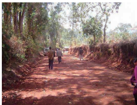
Side road of the construction site
