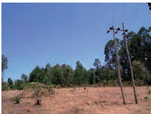
Power lines within the construction site
