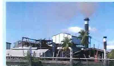
(Fuel for Fiji Sugar Cooperation boiler)
