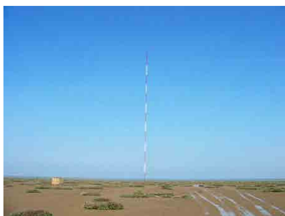
Overview of Wind Mast at Kuttikun Area
