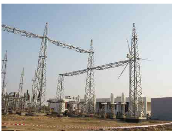
Grid Sub-Station for M/s Zorlu Wind Farm
