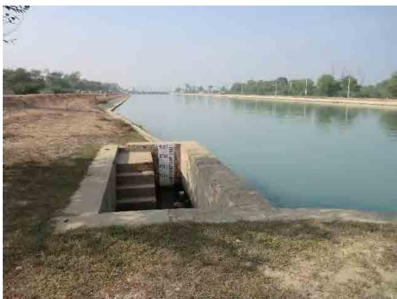
#2 Thal Main Line Upper W.L. Gauge (Nov.15, 2012)
