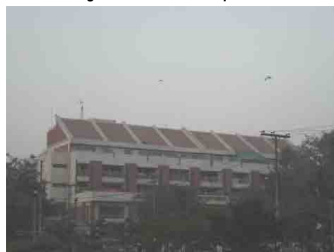
Figure 6-5: Photo from point 4
