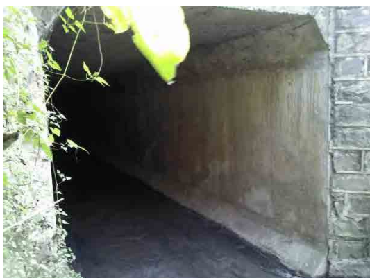
Box culvert of downstream side
