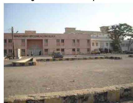
Figure 1-3: Photo from point 2
