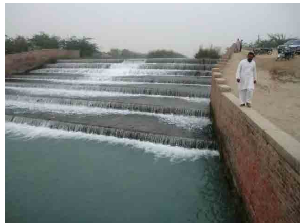
D/S Water Fall at Escape Channel of Thal Main Line Upper Canal (Nov.16, 2012)
