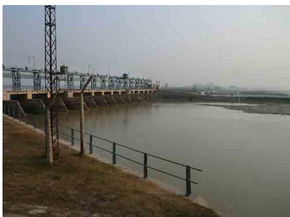
#485 (ADB-2) D/S of Existing Khanki Barrage (Chenab River) (Nov.14, 2012)
