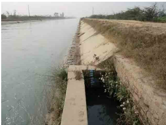
#5 Thal Main Line Lower RD 0+000 W.L. Gauge (Nov.16, 2012)
