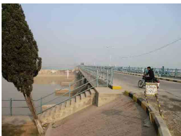
#597 (ADB-3) Quiderabad Barrage (Nov.12, 2012)
