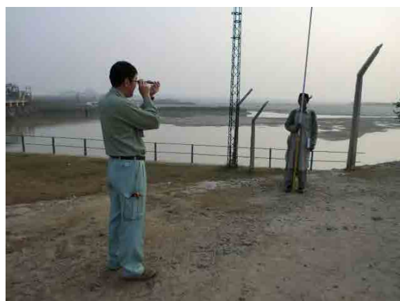
#485 (ADB-2) Leveling Survey at Proposed New Khanki Barrage Intake Site (Nov.14, 2012)
