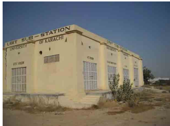
Figure 4-3: Photo from point 2
