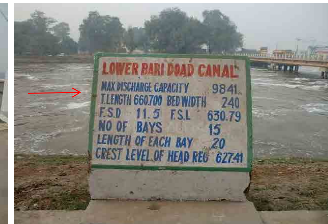
Lower Bari Doab Canal RD.0+000 (D/S)
