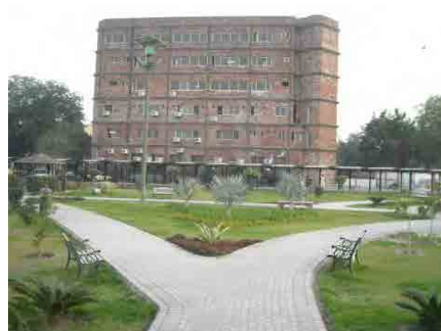
Figure 6-3: Photo from point 2
