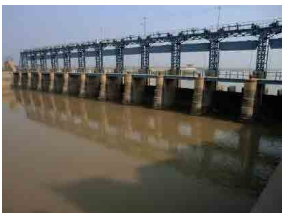
#485 (ADB-2) Khanki Barrage (Chenab River) Weir Length = 4,386ft = 1,337m (Nov.14, 2012)
