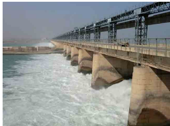
#2 Thal Main Line Upper RD 0+000 L = 1576.62ft = 480m (Nov.15, 2012)
