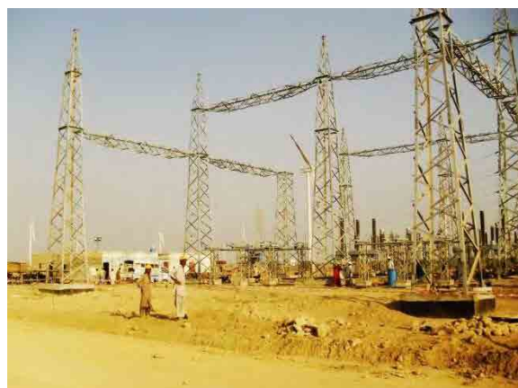
Under Construction of Grid Sub-Station for M/s Zorlu Wind Farm
