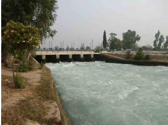
#5 Thal Main Line Lower RD 0+000 D/S Canal (Nov.16, 2012)
