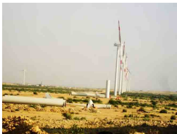
VESTAS Wind Turbines in Commissioning Phase
