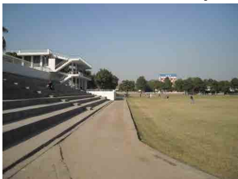
Figure 6-2 Photo from point 1
