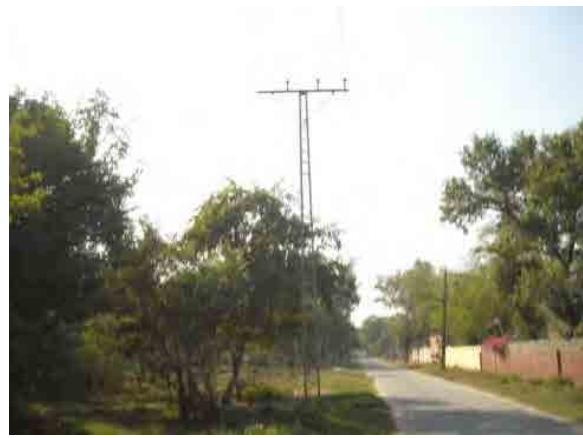
Figure 4-3: Photo from point 2
