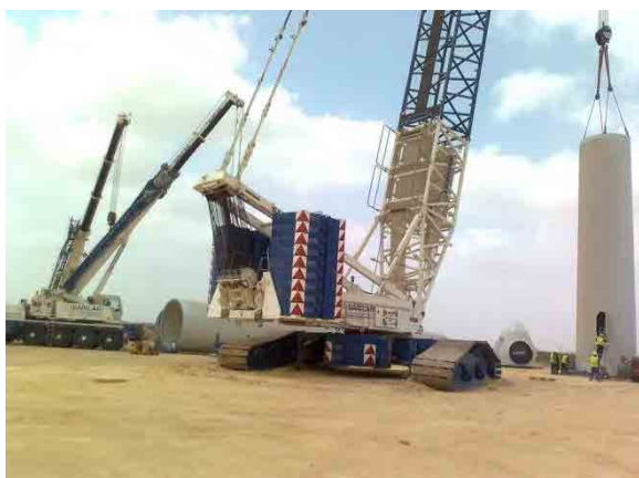
Wind Turbine Tower Erection at Site for VESTAS V90 1.8 MW
