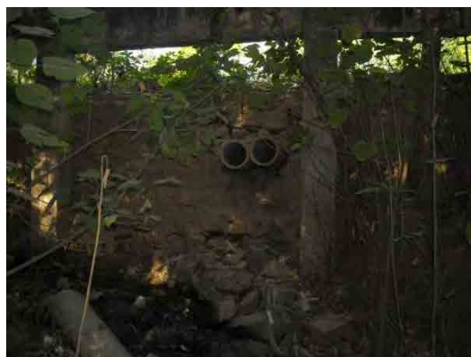
Pipes of road surface drainage
