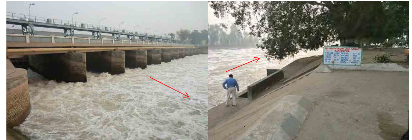
Balloki Sulemanki Link Canal RD.0+000 (from Right Bank)
