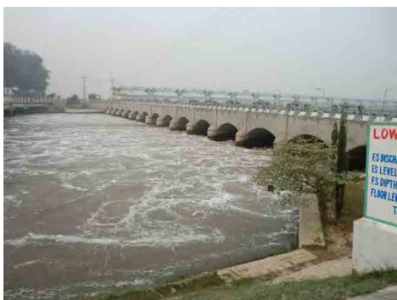
#643 Lower Bari Doab Canal (LBDC) RD 0+000 (Nov.10, 2012)
