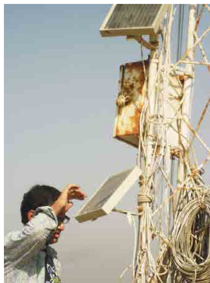
Wind Mast with Solar PV Panel and Data Logger
