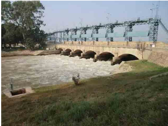
#490 (ADB-1) Lower Chenab Canal (RD 0+000) Main Regulator (Nov.14, 2012)
