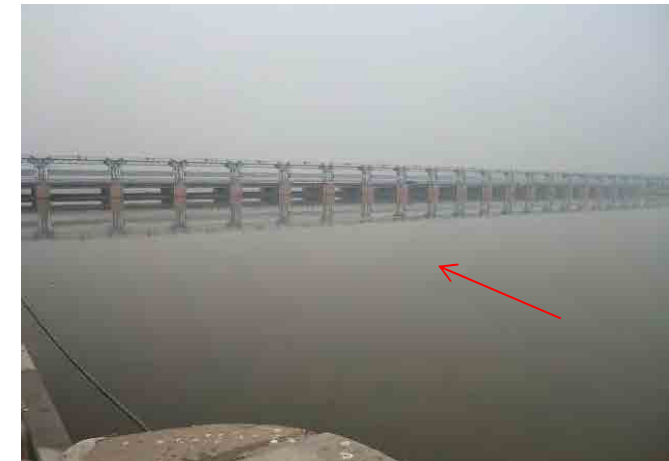
Balloki Headworks Upstream View (from Left Bank)
