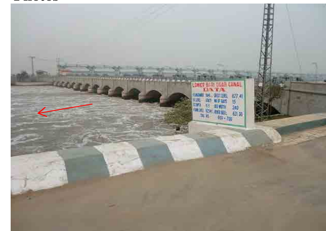
Lower Bari Doab Canal RD.0+000 (from Left Bank)
