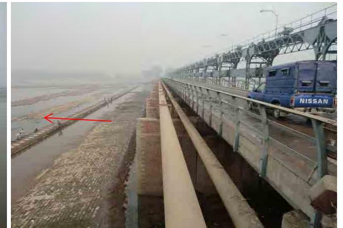
Balloki Headworks Downstream (from Left Bank)
