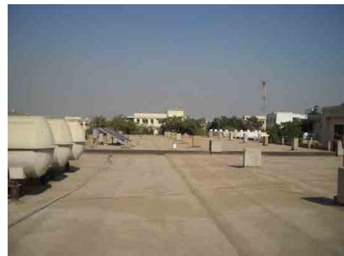
Figure 3-4: Photograph of roof top
