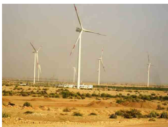
VESTAS V90, 1.8 MW Wind Turbine Generators
