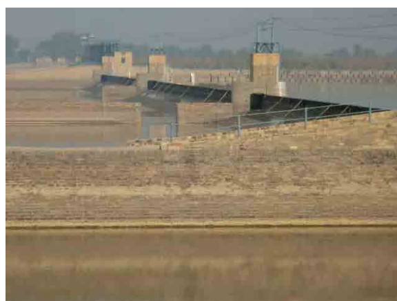
#485 (ADB-2) Khanki Barrage (Existing) (Nov.14, 2012)
