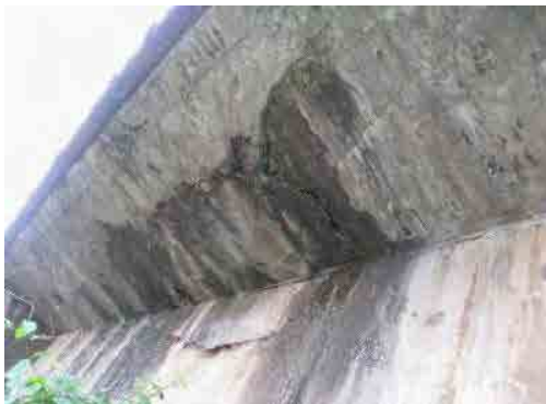
Photo-7 Repaired Portion
