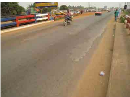
Photo-6 Condition of Surface (Downstream side)
