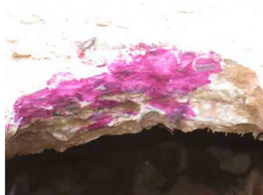
Photo 2 Test result at slab
