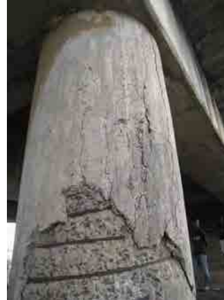
Photo-12 P-3, Downstream side (Upper)
