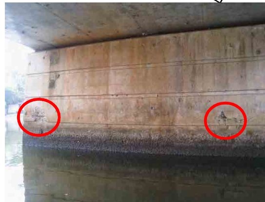
Photo-10 Status of Abutment (North Br., Free port side)
