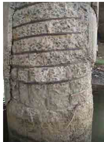
Photo-13 P-3, Downstream side (Lower)
