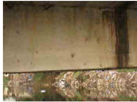
Photo-9 Damages by shot
