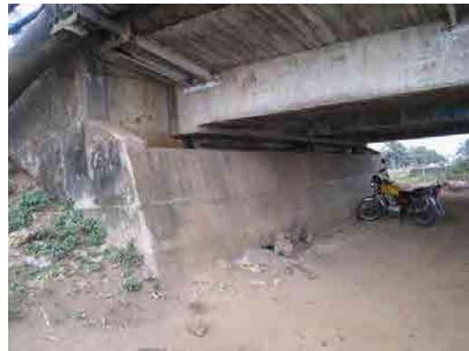
Photo-15 Abutment 1 (Free Port Jct. side)
