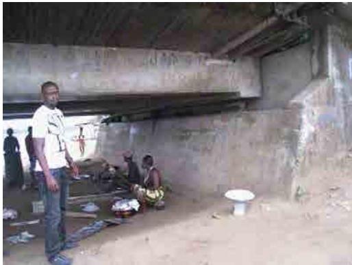
Photo-14 Abutment 1 (Free Port Jct. side)
