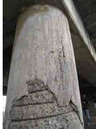
Photo-12 P-3, Downstream side (Upper)
