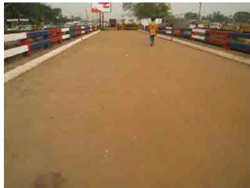
Photo-5 Condition of Surface (Upstream side)
