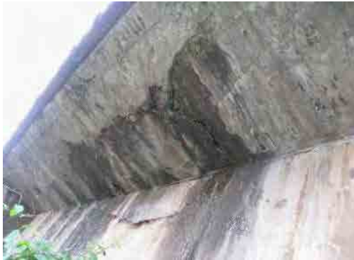
Photo-7 Repaired Portion
