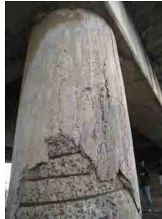
Photo-12 P-3, Downstream side (Upper)
