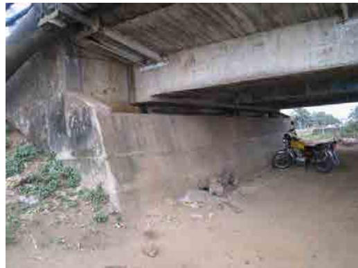
Photo-15 Abutment 1 (Free Port Jct. side)
