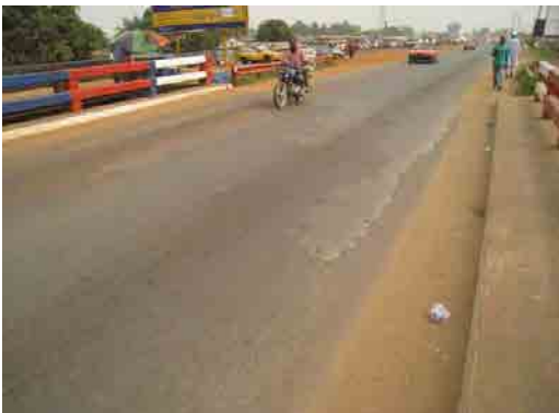
Photo-6 Condition of Surface (Downstream side)
