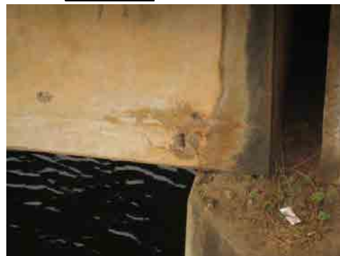
Photo-9 Appearing Reinforcement bar
