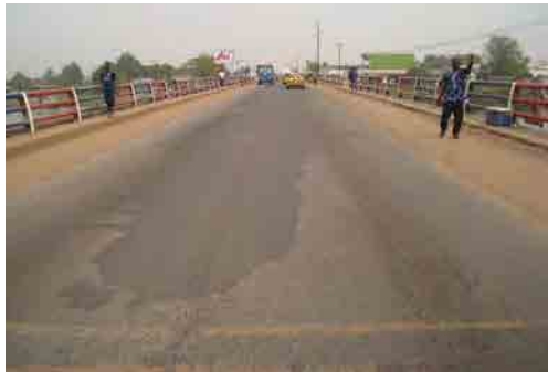
Photo-3 Condition of Surface
