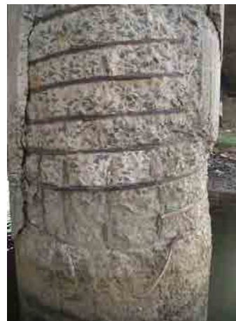
Photo-13 P-3, Downstream side (Lower)
