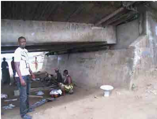
Photo-14 Abutment 1 (Free Port Jct. side)
