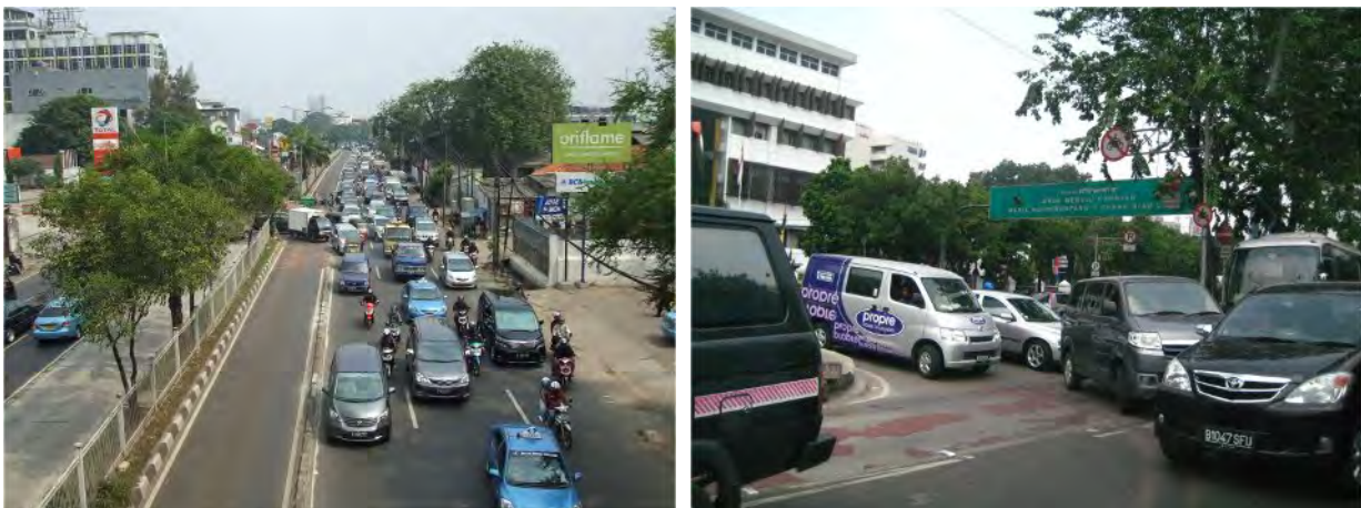
Transjakart – Bus lane is blocked by U-turn traffic Photo: Nippon Koei Co., Ltd.
