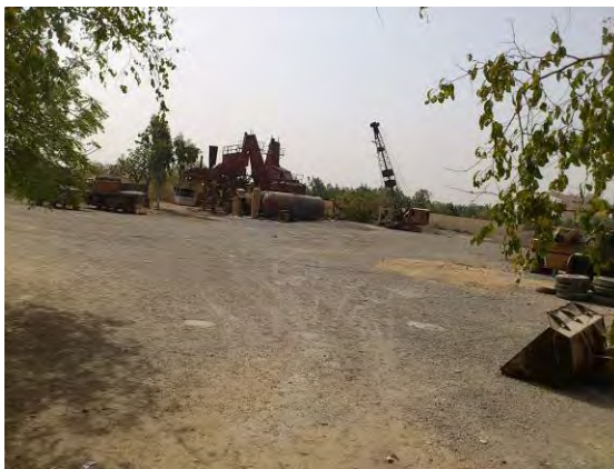
Existing Condition of Red Line Depot(2)
