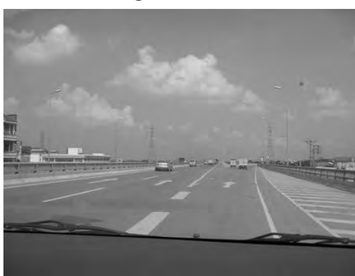
STA31+100 PhapVan Junction
