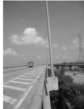
STA31+100 PhapVan Junction
