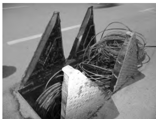
Cable Installation (VNPT)
