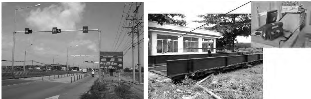
Figure 5.62 WIM System (Left) /Static Weigh System (Right) /Static Weighbridge (Below)
