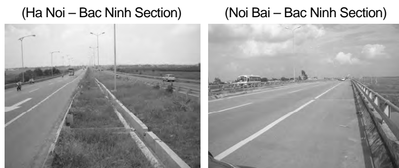
Figure 13 Existing Condition of Traffic in Northeastern Area of Ha Noi
