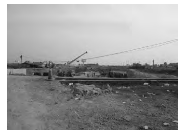
Earth Work of Noi Bai-Viet Tri
