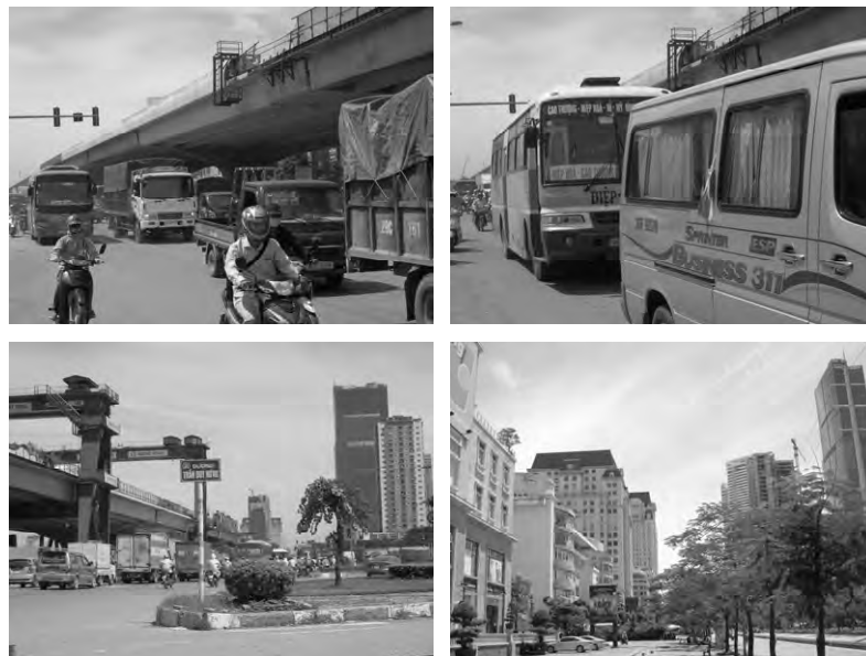
Figure 14 Existing Condition of Traffic in Southwestern Section of Ring Road 3
