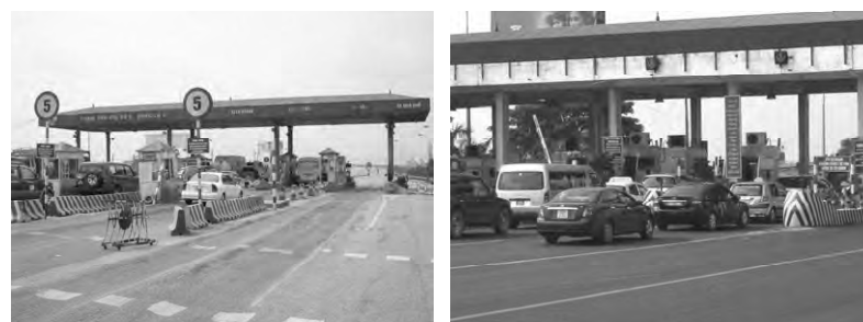
Figure 3.18 Existing Condition of Vehicle Queueing at Tollgate
