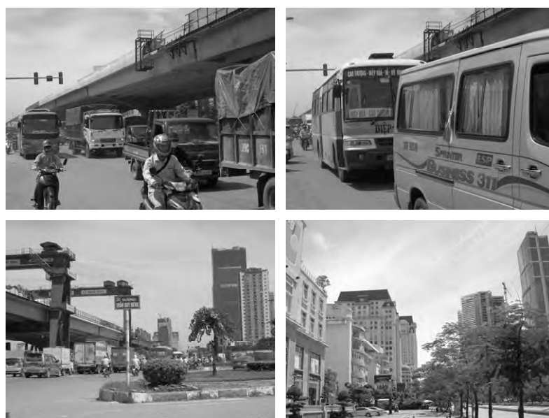
Figure 3.14 Existing Condition of Traffic in Southwestern Section of Ring Road 3
