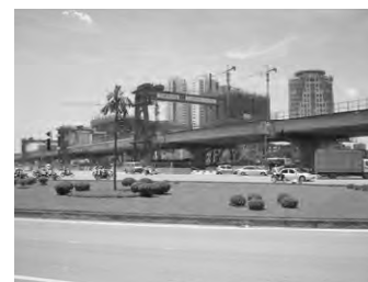
Viaduct on Ring Road 3 at Trung Hoa
