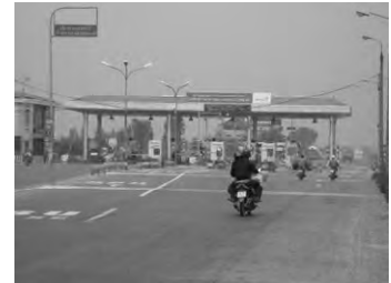
Tollgate at Cau Gie
