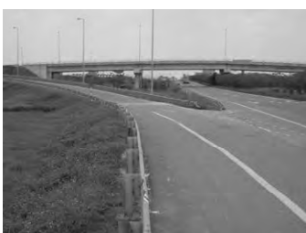
Bac Ninh Junction
