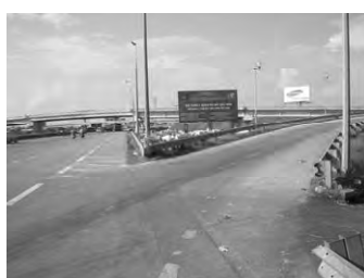
Noi Bai Interchange
