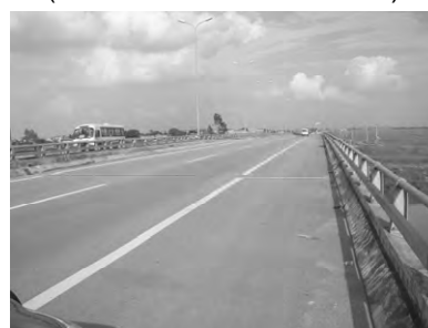
(Noi Bai – Bac Ninh Section)
