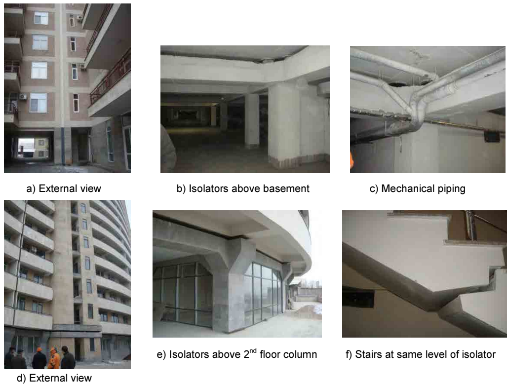
Figure 6.1-9 New residential buildings using seismic isolators in Yerevan
