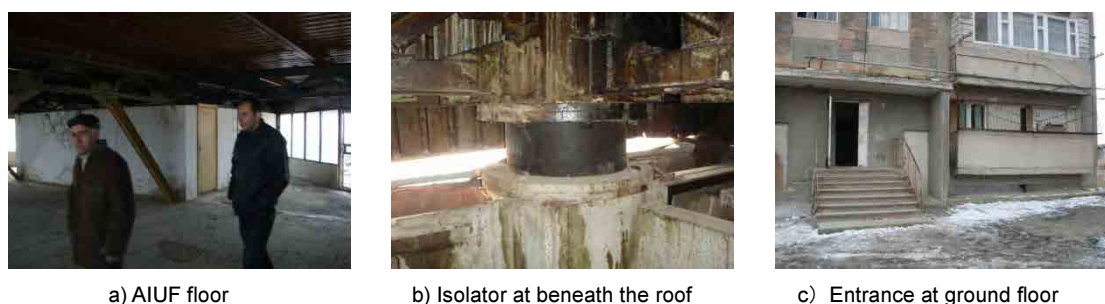
Figure 6.1-6 Retrofitting by Tuned Mass Damper (AIUF) at roof for frame panel (Series 111)
