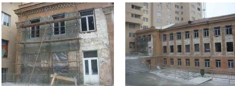
Retrofitting of school building (Mortar and wire-mesh jacketing on stone walls), Kentron No.29.
