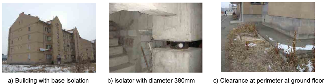
Figure 6.1-10 Residential buildings with seismic isolation at Gyumri
