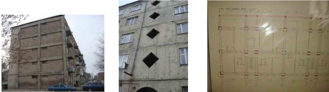
Figure 6.1-3 Retrofitting of damaged stone building (series 1-451),
