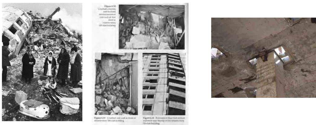
(left) Collapsed 10-story 'lift slab' at Gyumri (provided by NSSP EEC)
