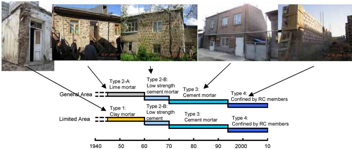
Figure 5.1-16 Proposed structural category and supposed constructed year
