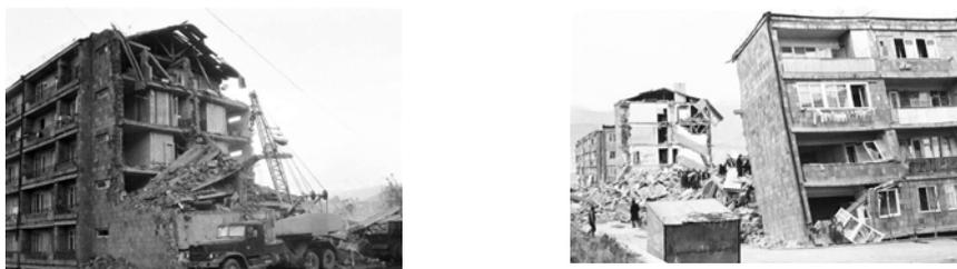
(a) Collapse of side portion at Gyumri (by NSSP EEC) (b) Collapse of center portion at Gyumri (by NSSP EEC)
