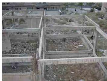
Figure 5.1-11 Badalyan type under construction
