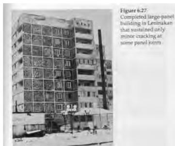
Figure 6-27 Completed large-panel building in Leninakan that sustained only minor cracking at some panel joints.
