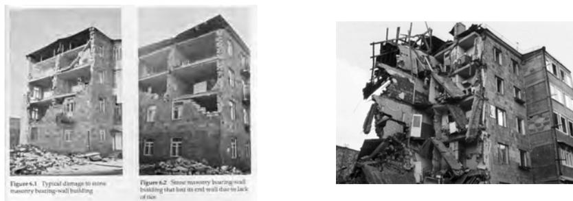
(a) Out-of-plane collapse of stone walls (ref. 1) (b) Partial collapse of building at Gyumri (by NSSP EEC)
