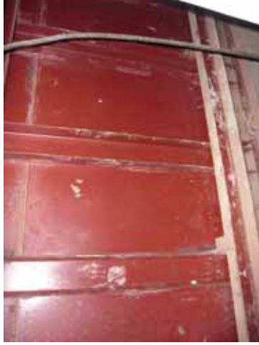
Outside of flocculation basin (upstream)
