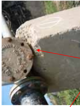
Damage by Scraping
