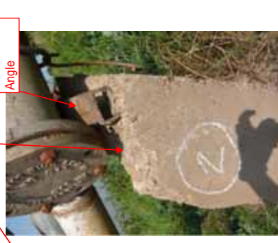
Damage by Scraping
