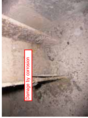
[Post in bottom of sedimentation basin (Brock 1)]
