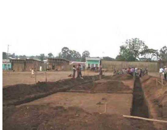
Trench excavation for foundation (16 Mar. 2011)
