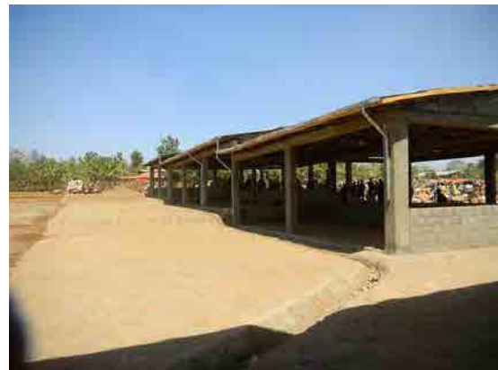
Overview of Block 1 (02 Feb. 2012)
