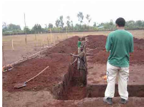
Trench excavation for foundation (15 Mar. 2011)
