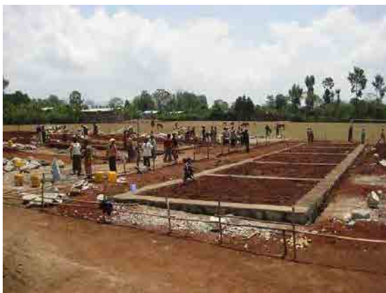
Masonry foundation works (07 Apr. 2011)
