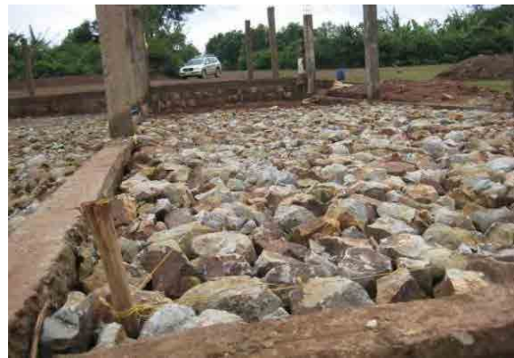
Hard core for floor slab (20 May 2011)
