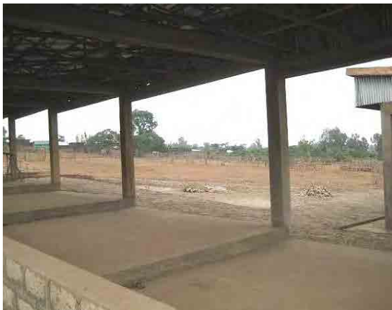
Inside situation after roofing (30 Jun. 2011)
