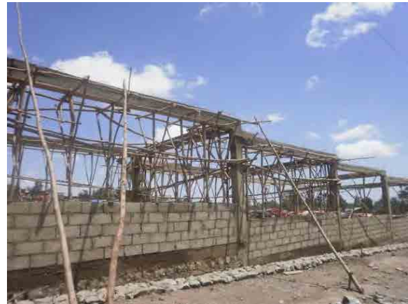
Roofing works (05 May 2011)
