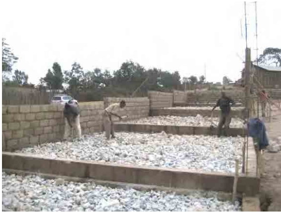
Stone hard core and block works (05 Apr. 2011)
