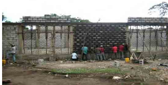
Block and top tie beam works (09 June 2011)
