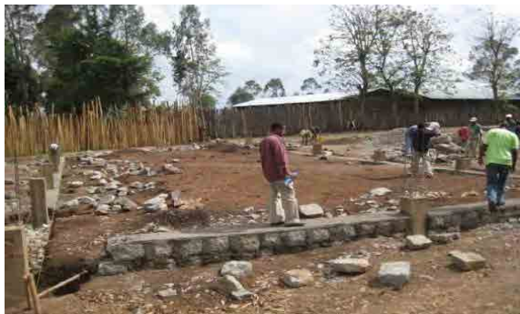
Masonry foundation works (07 April 2011)
