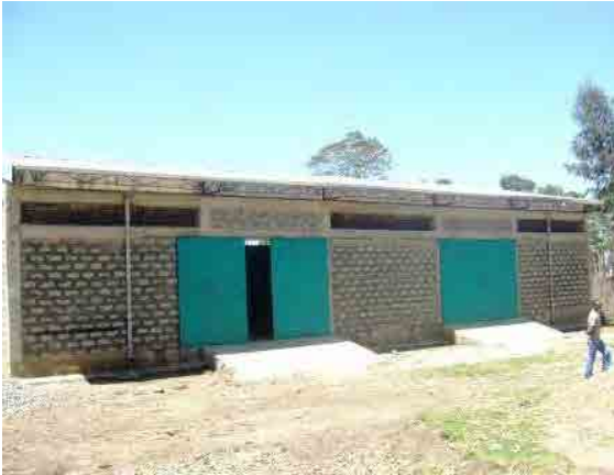
Warehouse of Angacha Union constructed with the technical and financial support of SAMS-SNNPR (PP08)
