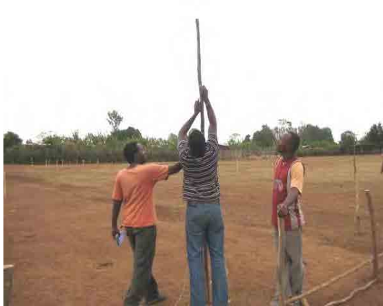
Survey and staking out (03 Mar. 2011)
