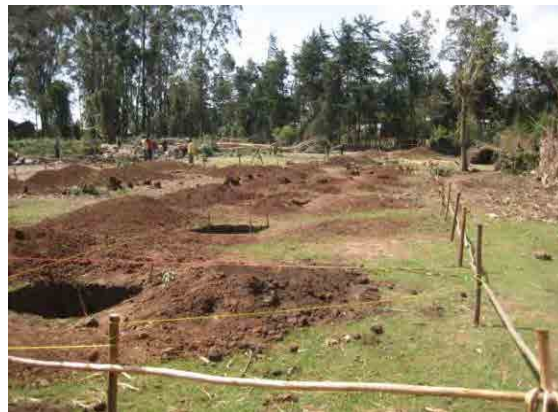
Foundation excavation (23 March 2011)
