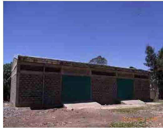
General view after completion (21 Oct. 2011)
