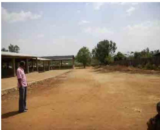
Backside of Block 1 : No trader uses booth (29 Feb. 2011, on a market day)
