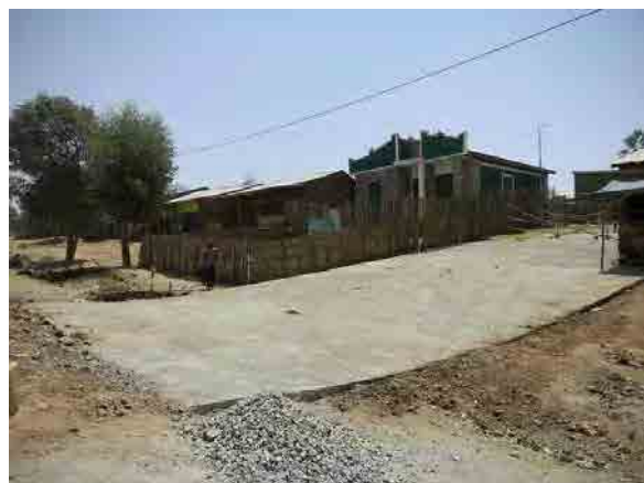
After completion of ford type ditch crossing structure (09 Mar. 2012)
