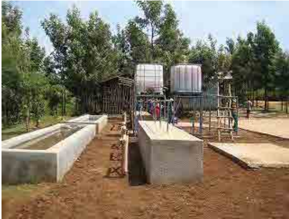
Constructed washing facility
