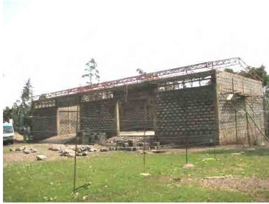
Roofing works (08 July 2011)
