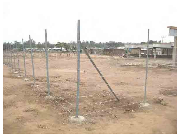
Fencing works (11 Jul. 2011)
