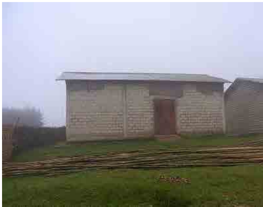
Abala PC (Hulla woreda) has two warehouses with ventilation openings, built about 20 years ago, still under-utilized. The capacity is about 200 tons each.
