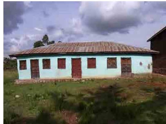
Bonoya Chire PC (Boricha woreda) owns this warehouse. Stores maize and haricot bean.
