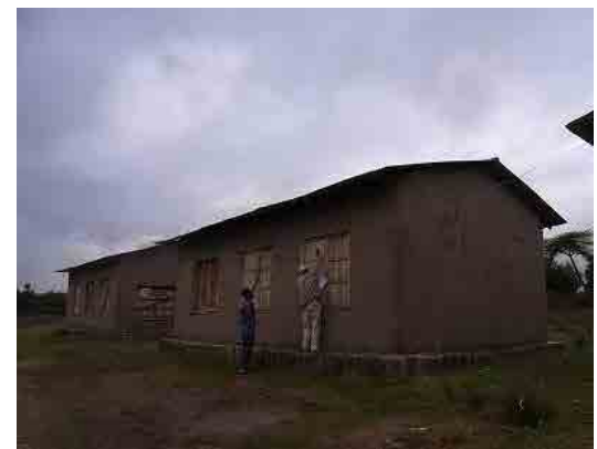
Hantatena PC (Lokko Abaya woreda). Both 2 warehouses with 1 door and 6 windows that are rented from Kebele Municipality.
