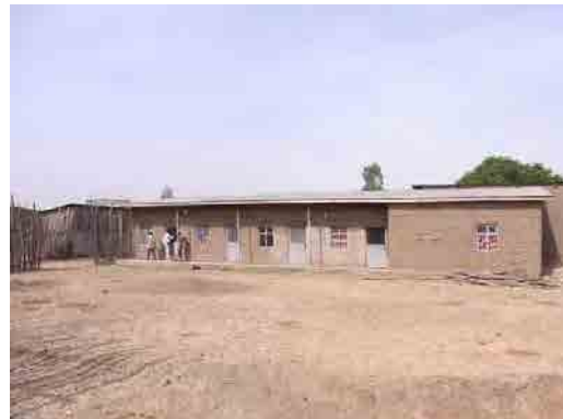
Office houses are used as warehouses
