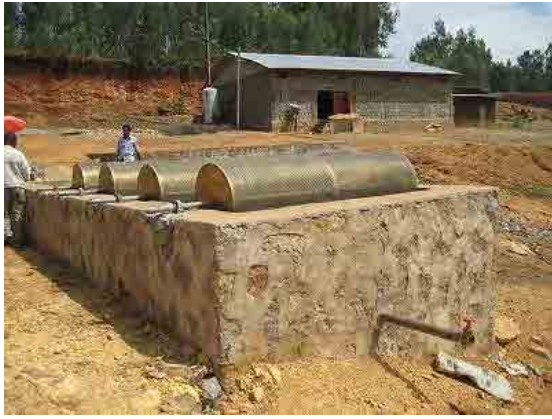
Newly built facility
