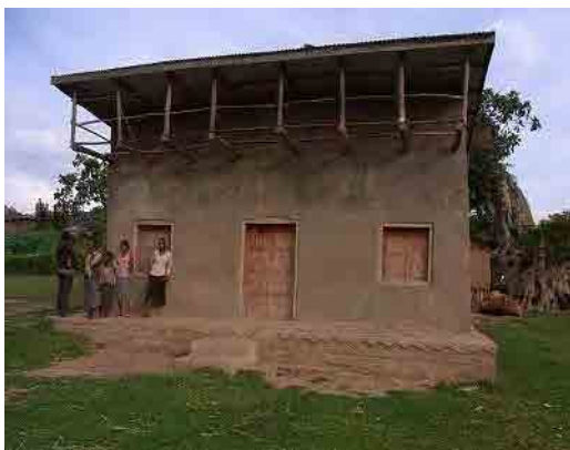
Shello Balela PC (Boricha woreda) has rented this kind of warehouse from individuals.
