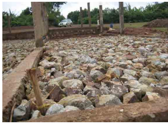
床下栗石工事 (20 May 2011)
