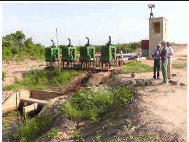
Prairie Volta Farm River water pumped up from the Volta river again lifted up to the paddy field by similar engine pumps.
