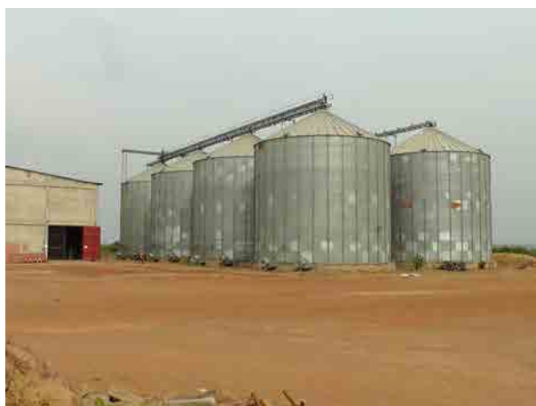
Prairie Volta Farm Storage silos of the Prairie Volta Farm in Aveyime The silos have total capacity of 30,000m 3 . The silos are available to store the produce of NDIS.
