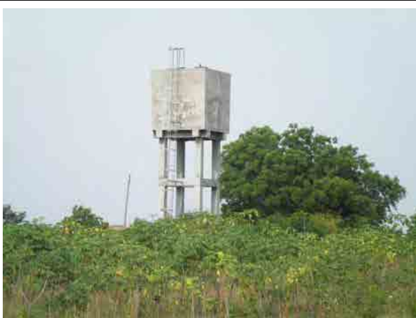
Elevated water tank Water is supplied to the villages through the elevated water tanks.
