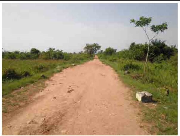
Road in the command area Gravel and sand materials is strong enough for traffic. Drainage ditch is also necessary to protect road surface.
