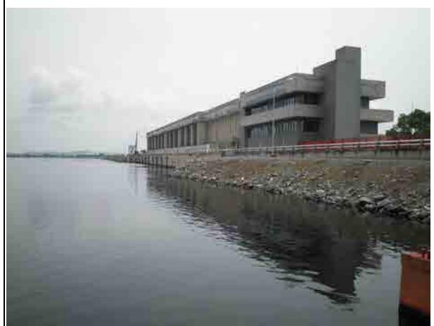
Hydraulic plant of the Kpong dam Power plant is located at the center of the dam. Power units are installed below the control house.
