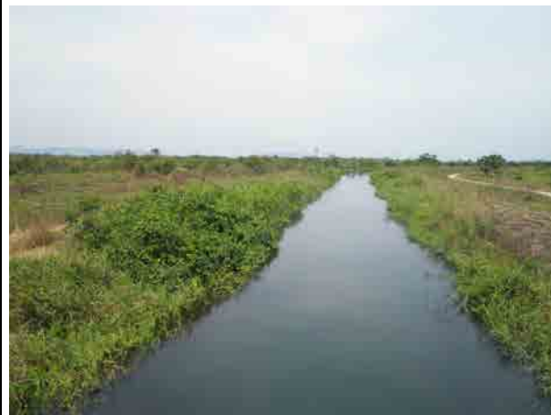
KIS Akuswe Canal Canal section about 4km downstream of the intake. OM road is well maintained.
