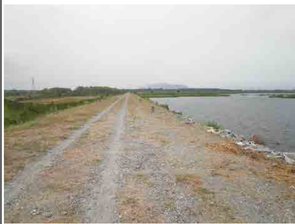
Right side of the Kpong dam Intake of NDIS is proposed at far right side the photo.
