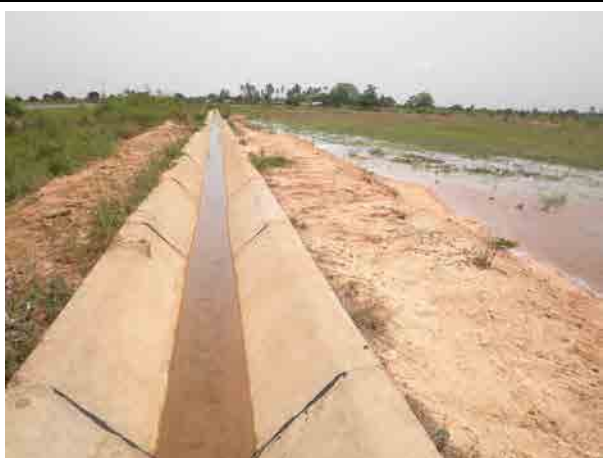
Irrigation canal in Aveyime Irrigation project Canal surface was lined with concrete. Land preparation water was supplied to the paddy. Land leveling work was completed.
