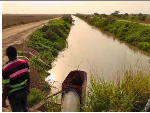
Prairie Volta Farm Irrigation canal in the paddy field Irrigation water pumped up from the Volta river is diverted through the irrigation canal.
