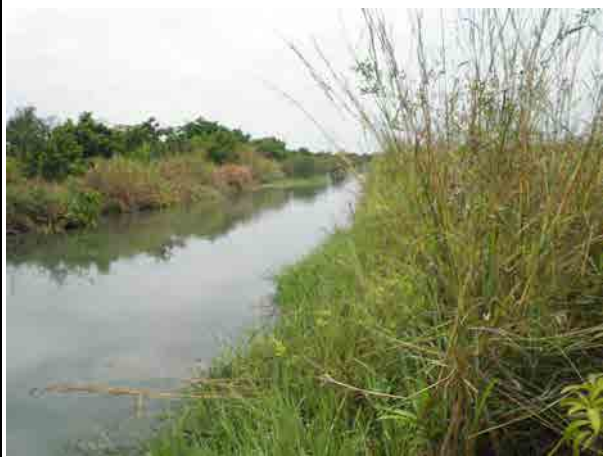
KIS canal (Akuse Main Canal) About 14 km downstream of the intake. Canal bank is covered in weeds. Periodical weeding work is carried out by the project office.
