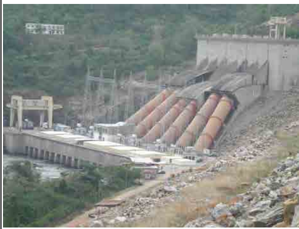
Hydraulic plant of the Akosombo dam located at upstream of the Kpong dam. One penstock has a flow capacity of 200 \text{ m}^3/\text{sec} .
