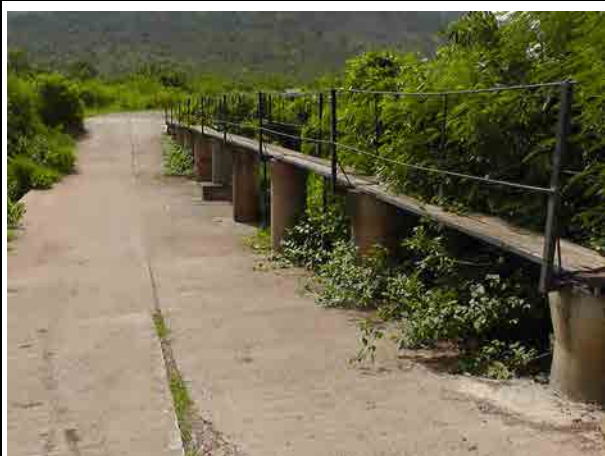
OM road crossing the drainage channel Vehicles are passable in the water depth of about 0.3m during the rain. Pedestrian bridge is shown in the right of the photo.
