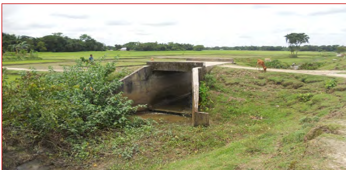
Image 2 Overview of Goatola portion of proposed bridge construction site
