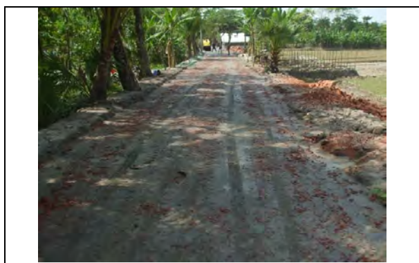
District: Pirojpur, UZ: Mothbaria, Pkg: PIROJ-07 AS in progress
