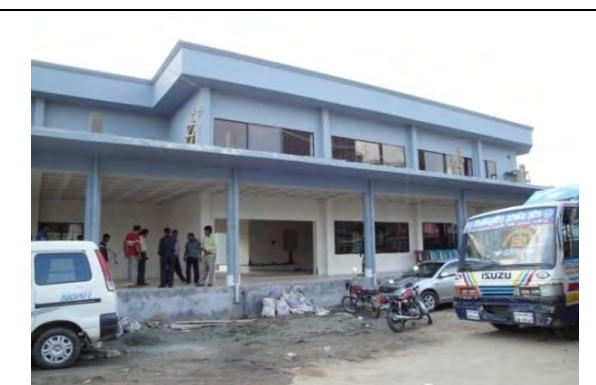
Gazipur Bus Terminal
