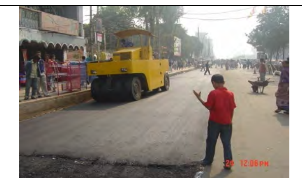
Bangabandhu Road in Narayangonj Pourashava
