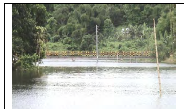
Foot Bridge in Rangamati
