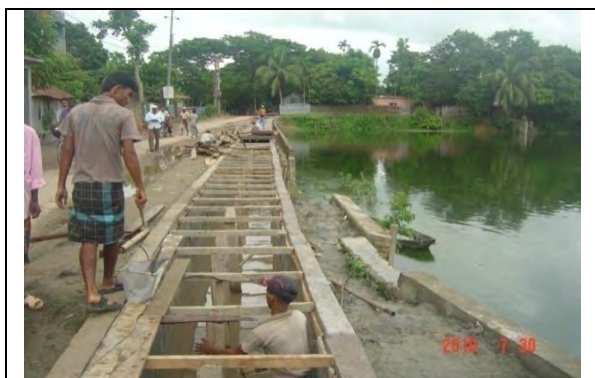
Drain Construction in Laksham Pourashava
