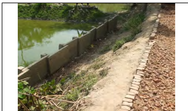
District: Barisal, UZ: Hizla, Pkg:-02 Double plate palisading work
