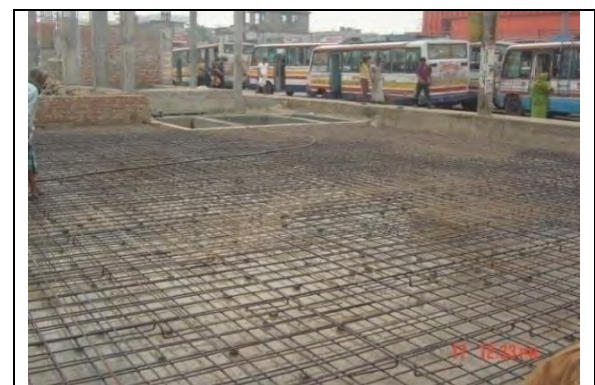
Chapai Nawabgonj Pourashoba Bus Stand Construction Work
