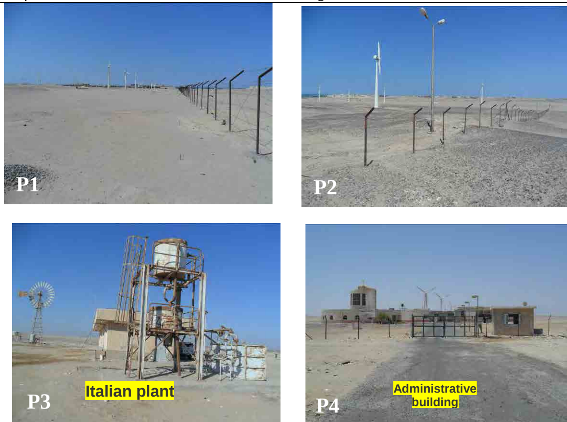
Figure (6) Wire fence and some structures near the project area
