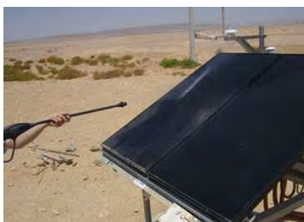
Fig. 5-2-3 Cleaning method by high pressure water sprayer
