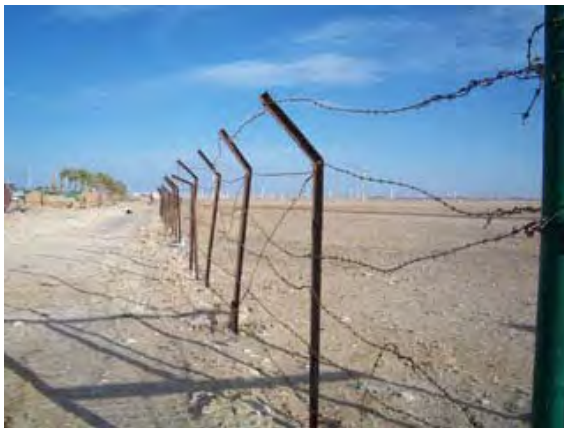
Photo 3-1-1-11 Existing site border fence (11)
