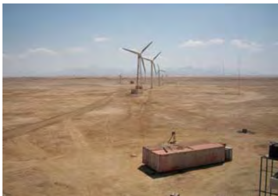
Photo 3-1-1-3 300kW and 100kW Wind turbine in the candidate site (3)
