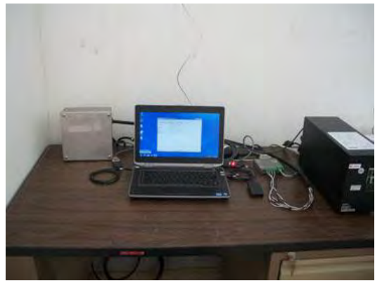
Photo 3-2-1-2 Inside view of Equipment
