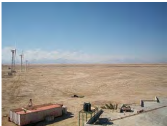
Photo 3-1-1-1 Site condition (northern-side)(1)
