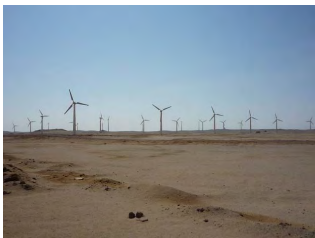
Photo2-2-3 Hurghada wind park (WINCON type)
