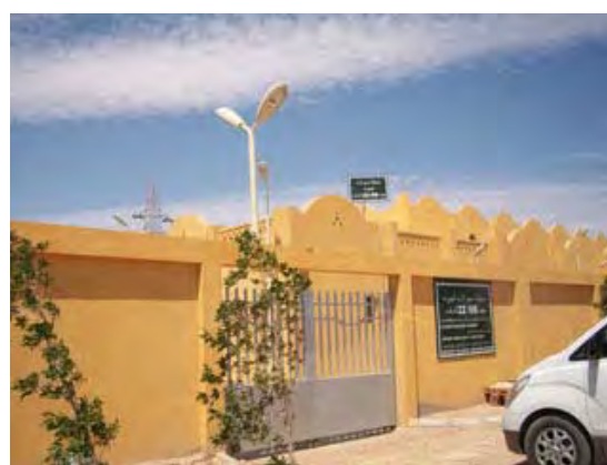
Photo 3-1-2-4 El-Gouna substation / Private sector (not energized yet)
