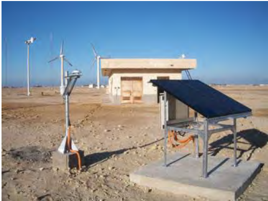
Photo 3-2-1-1 Outside view of Equipment
