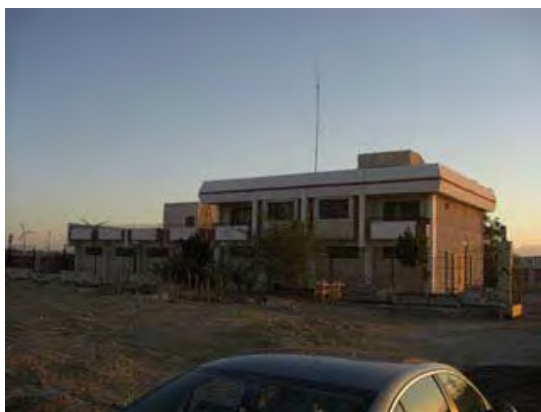
Photo 3-1-2-1 Hurghada wind Distribution Point
