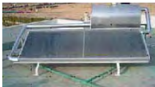
Photo2-2-7 Solar water heater Medical center: 2008 Source: Annual Report of NREA 2009/2010
