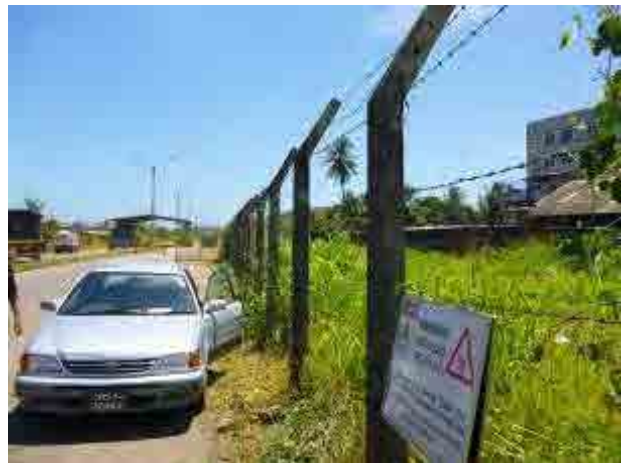
Port Access Road in Planned Route of New 220 kV Kelenitissa - Port Transmission Cable Line
