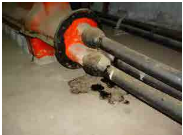
Existing 132 kV OF Cable Condition for Colombo E GS
