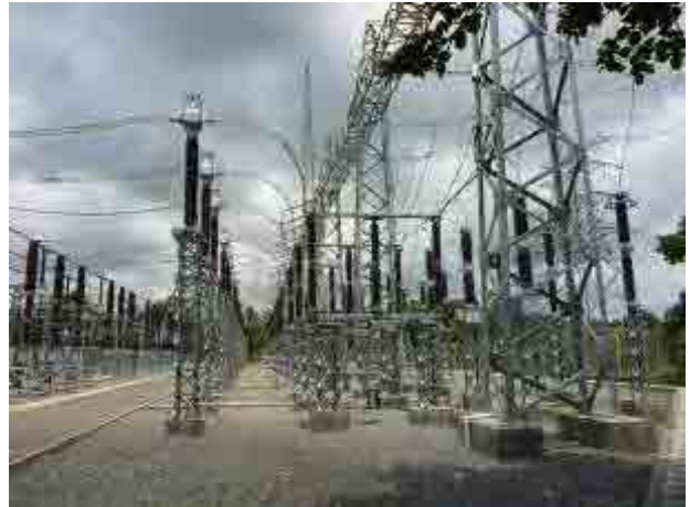
Extension Planned Area of 220 kV Switchyard at Veyangoda GS
