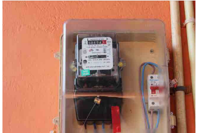
Electro-mechanical Energy Meter for Small Consumer
