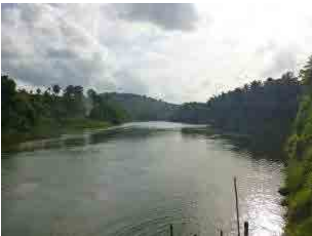
Crossing River in Planned Route of New 220 kV Veyangoda - Padukka Transmission Line
