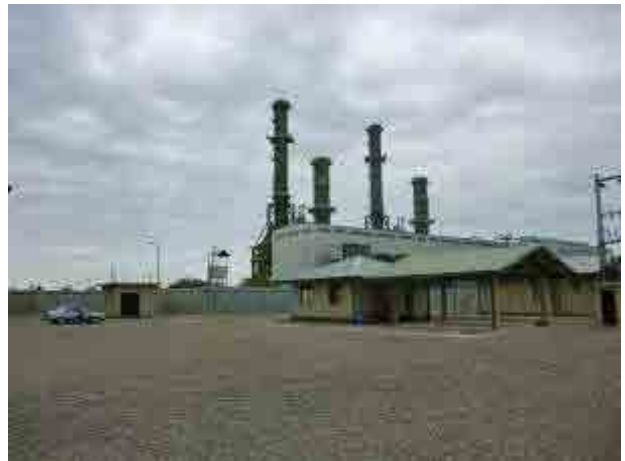
Extension Planned Area of 220/33 kV 2 x 35 MVA Transformer at Kerawalapitiya GS
