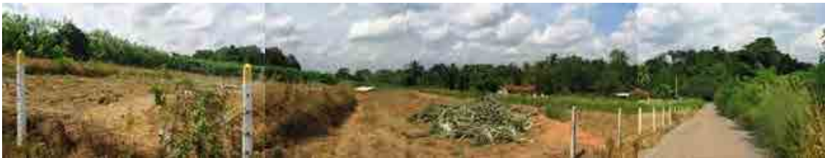
The land is identified as the site for Kirindiwela Switching Station. Chena cultivation is implemented and housing scheme is on-going.
